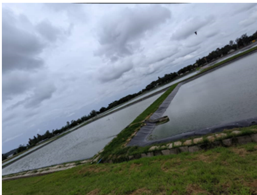
Butuja treatment ponds for connected pit latrines on the project area
