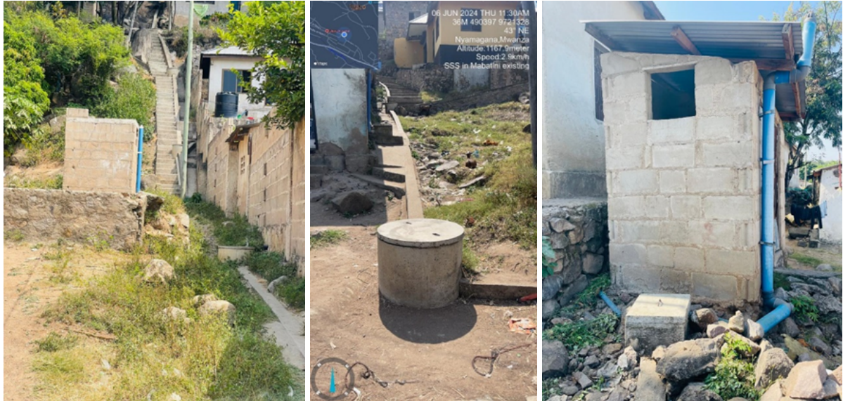
Existing simplified sewer system from connected pit latrines
