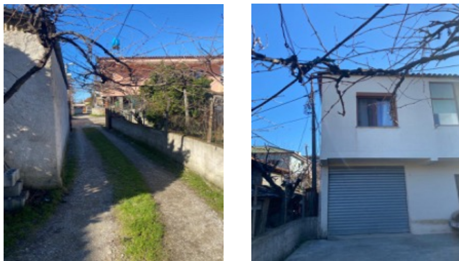
Figure 5-3 Structure used for business activity
