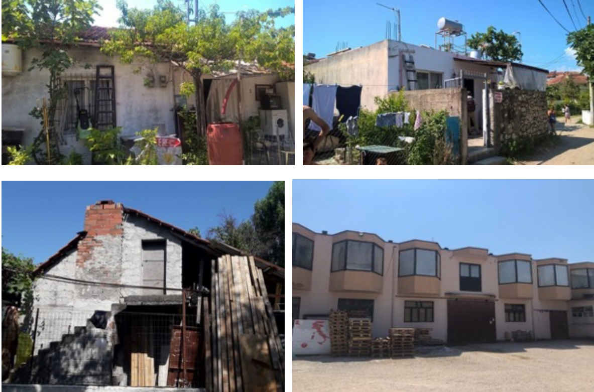
Figure 1-2 Example structures in the affected area (residential and nonresidential)
