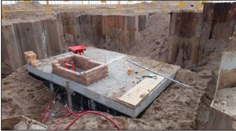
Figure 14. Example of BMH infrastructure. Source: AFR-IX Telecom.
