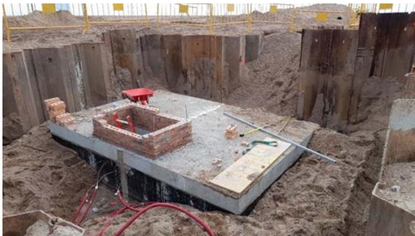
Figure 10. Example of prefabricated BMH infrastructure. Source: AFR-IX Telecom.
