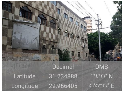
Figure 4-12: The mosque from outside (first mosque)
