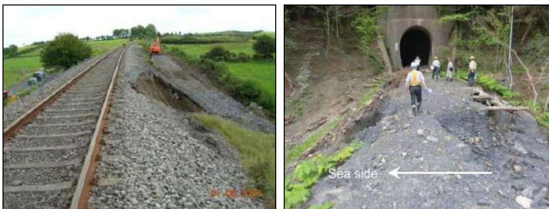
Figure 192 Erosion of the embankments before entering the tunnel - a potential threat to the safety of the railway traffic 41
