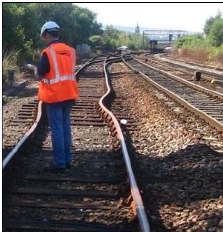
Figure 191 Bending the rails as a result of high ambient temperatures 40
