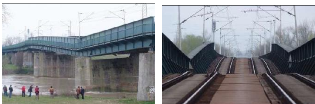
Figure 193 Bridge scouring and effects (Zagreb, 2009) 42
