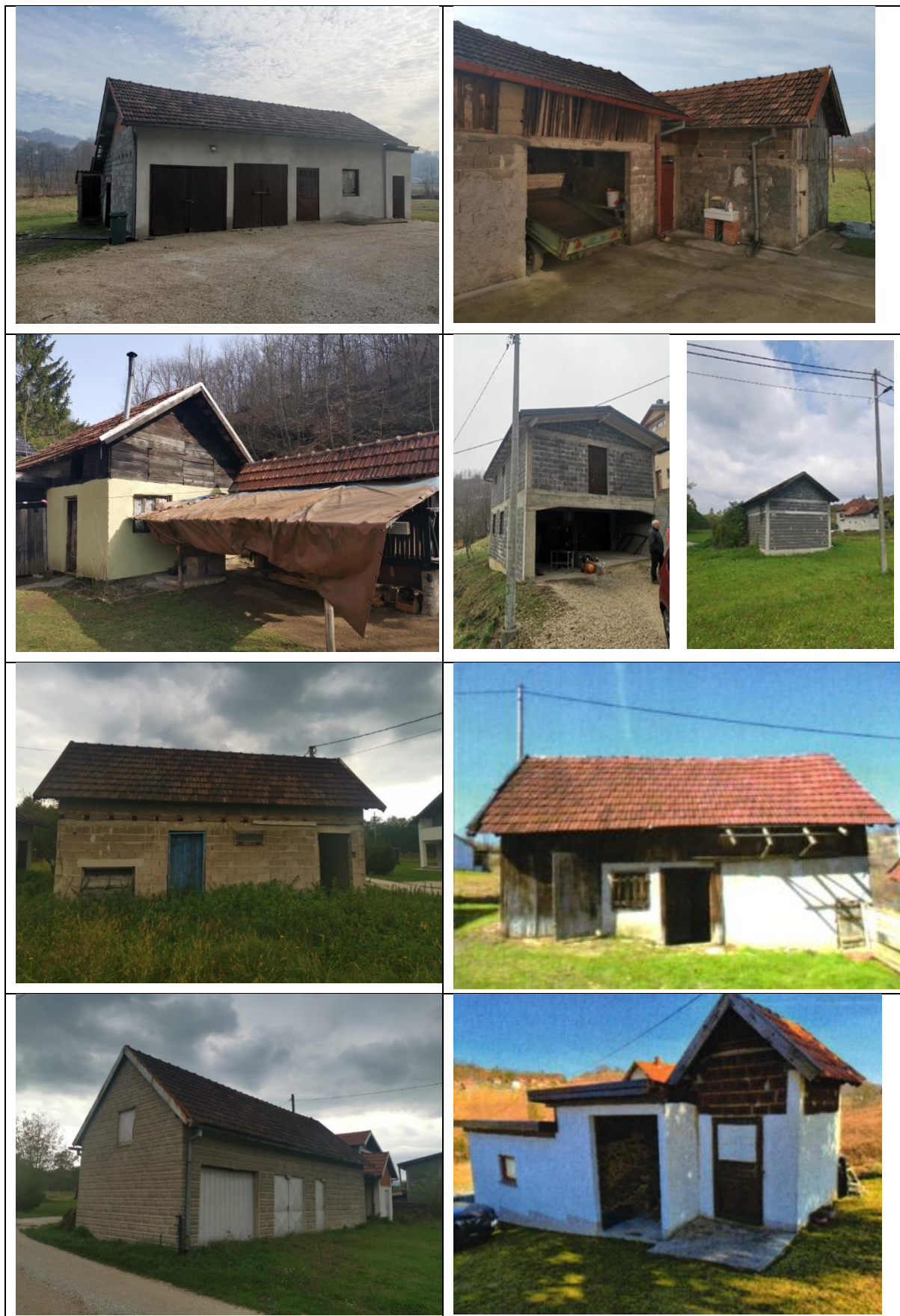
Figure 12: Pictures of some auxiliary structures affected by expropriation
