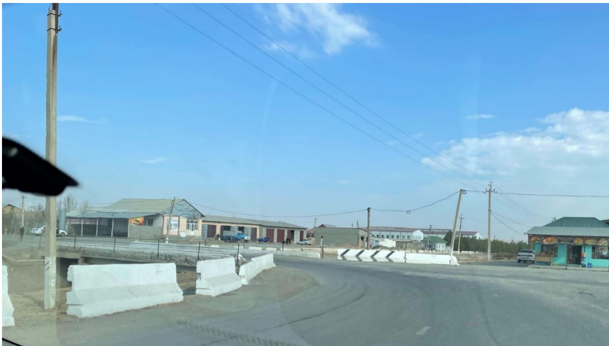
Figure 6-54. Pinch point on minor road to Karakchi
