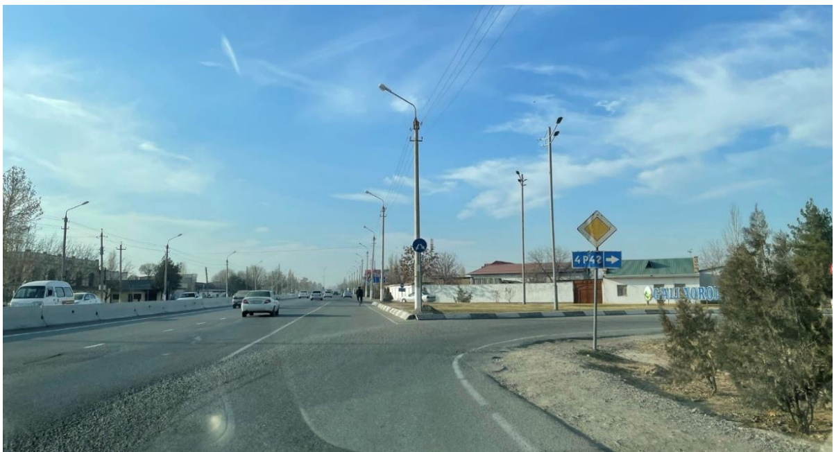
Figure 6-52. Junction from M39 at Gallaoral onto Minor Road (4P42) to Karakchi
