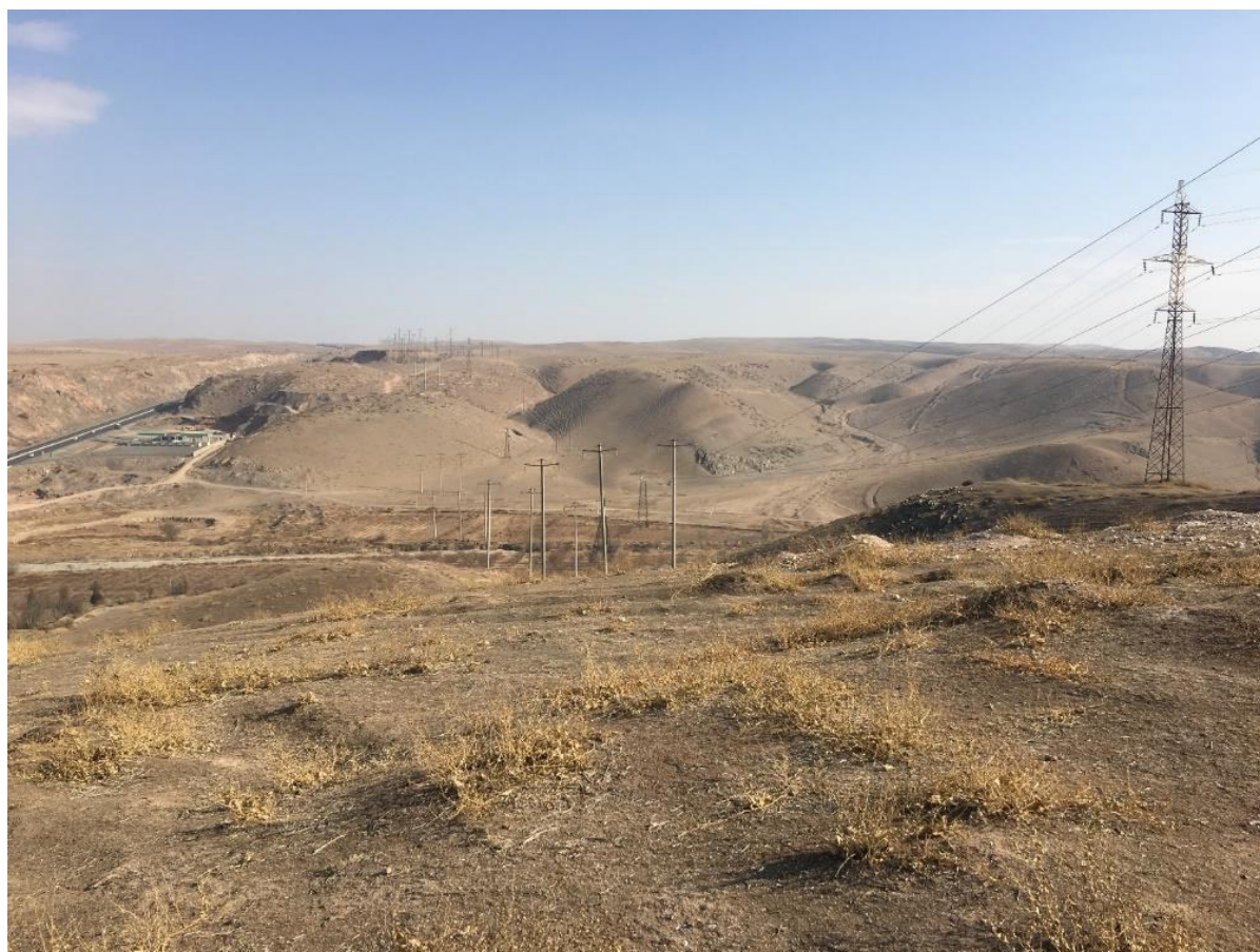
Figure 6-29. View across to the foothills for the Overhead Line between the Sanzar river valley and the existing Saribazar substation – Capparis spinosa sub-shrub punctuating the degraded pasture in the foreground
