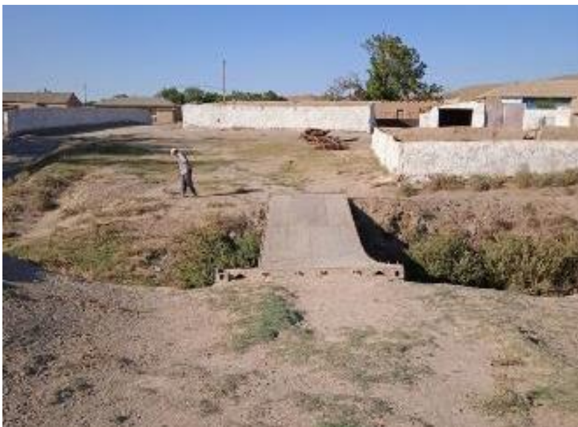
Figure 6-48. Small bridge to primary School 54 in Chayonli village
