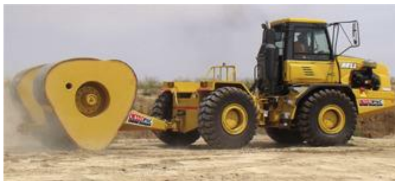
Figure 2-14. Rolling dynamic compaction (RDC)
