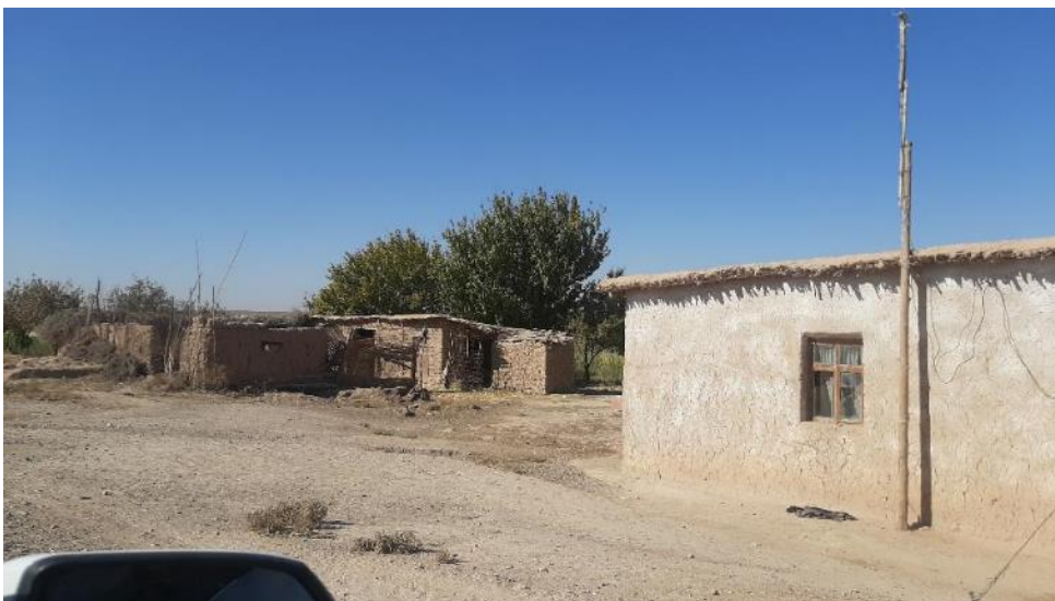
Figure 3-12. A house South of the Project Site
