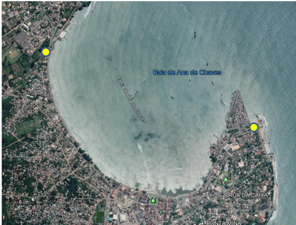
Figure 5 Aerial view of the Section 2: Ana Chaves Bay. Ch. 2+760 – 5+900
