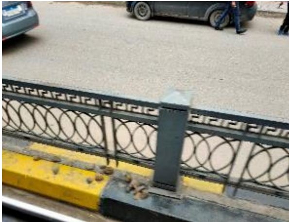
Figure 4-80: Fence close to Raml station
