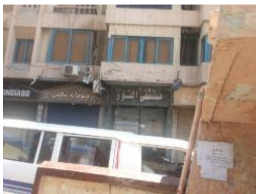
Figure 4-25: El Nor Hospital
