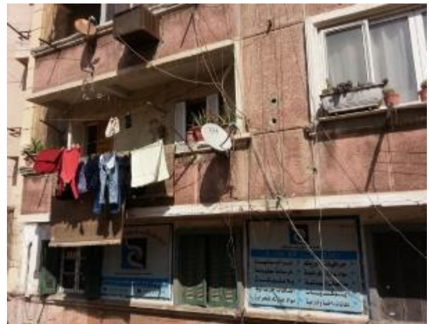
Figure 4-55: Buildings close to the tram fence
