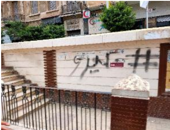
Figure 4-82: Concrete constructed fence
