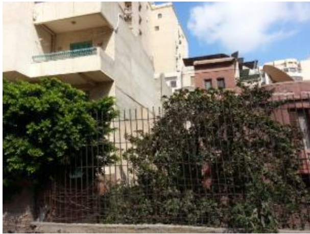
Figure 4-52: Newly constructed buildings
