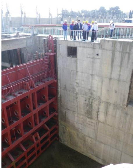
Picture 1 – One of the gates to be replaced
