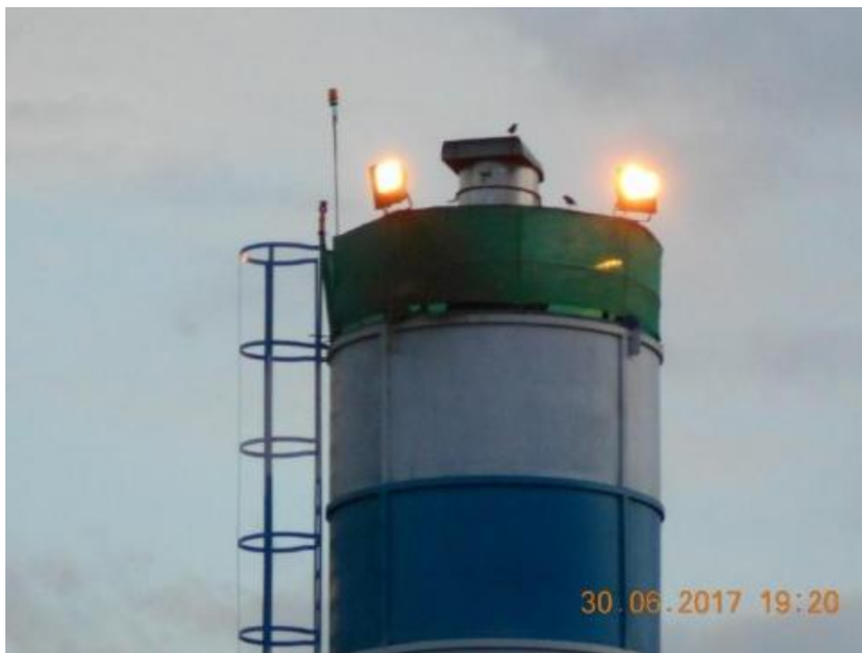
Figure 9.1. Silo top Aero Filter
