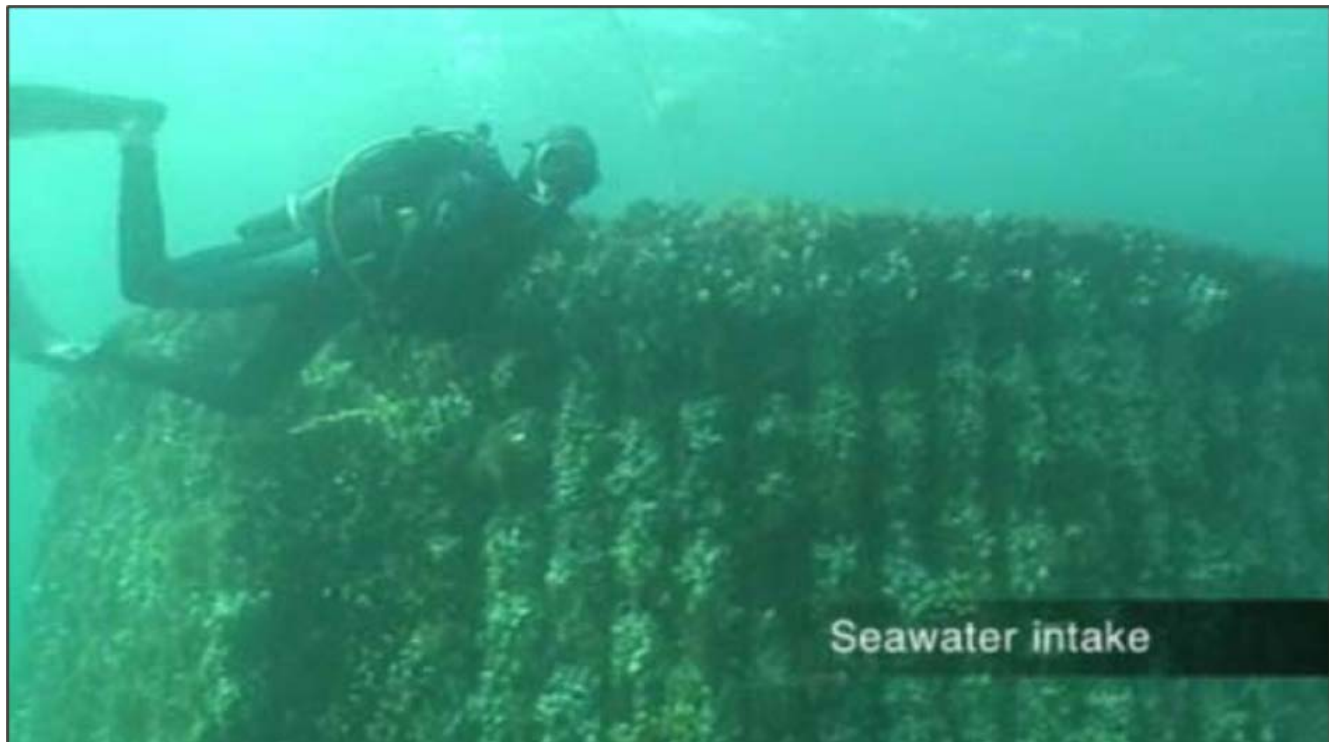
Figure 2-7: Macrofouling on screen of Intake Tower at Perth 1 SWRO plant
