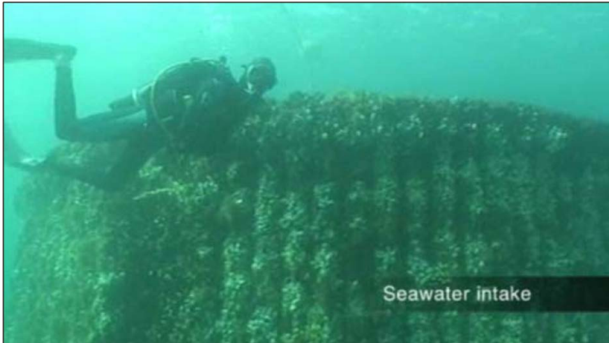
Intake Tower Screen Fouling Needs Cleaning by Divers (Perth SWRO)
