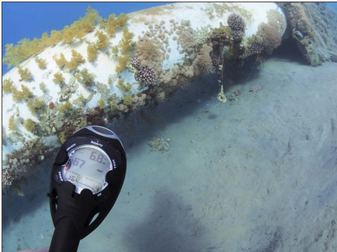
Figure 2-3: Gas Pipeline Observed by ESIA Team Divers
