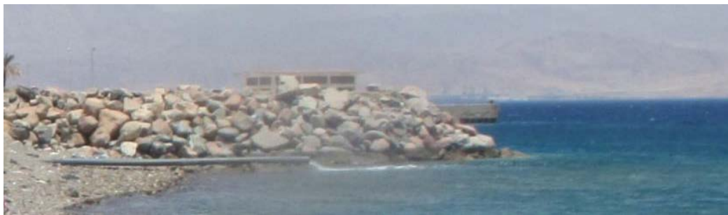
Figure 8-6: Taba SWRO Shore Brine Outfall Next to Rock Jetty
