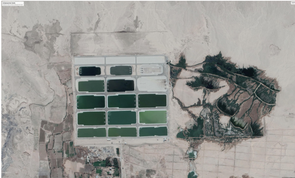
Figure 10: Non-functioning WWTPs in Sohaq and Assiut
