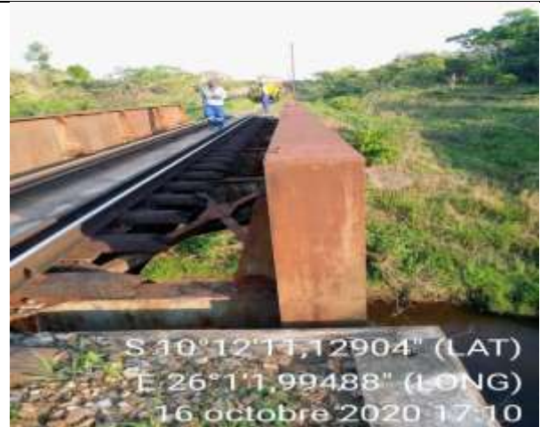
Photo . Pont Kafwa 13,22 m
