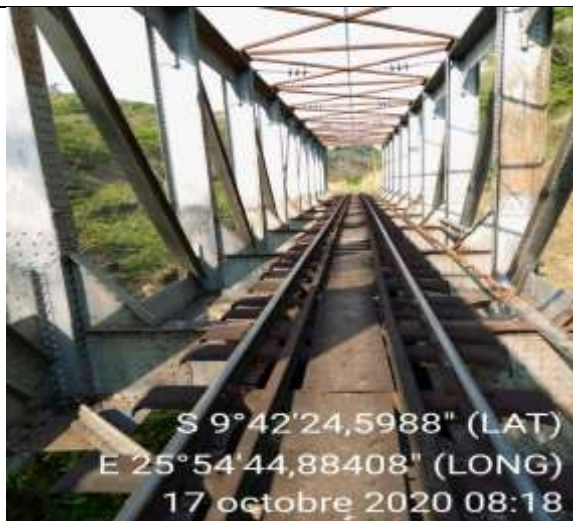
Photo. Pont Kafwa 30 m
