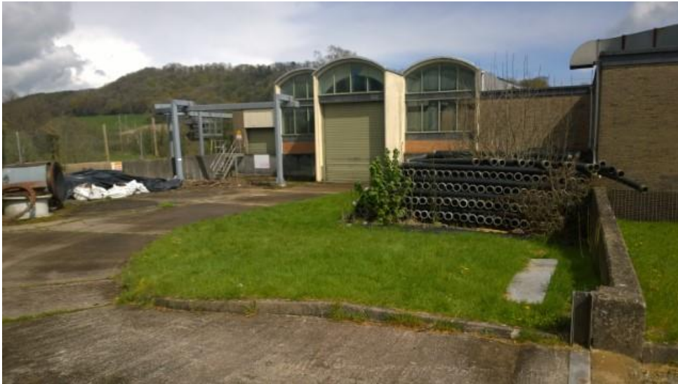
The Existing Raw Water Pumping Station
