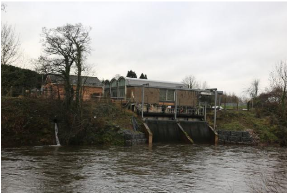
The Existing Raw Water Pumping Station Viewed from the River Usk
