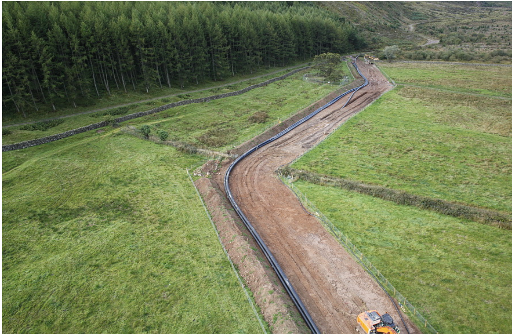
Example of open cut trench and pipe laying on United Utilities' South Egremont Scheme
