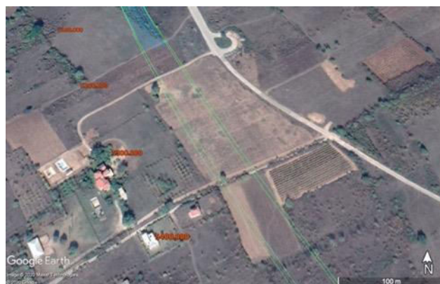
Figure 78: Houses in close proximity to the motorway in settlement Kosor (chainage 5+300 to 5+400)
