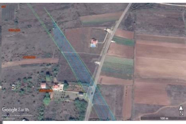
Figure 79: Houses in close proximity to the motorway in settlement Kosor (chainage 5+700)
