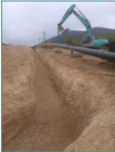
Figure 2: Construction phase of a pipeline (descent of the pipeline)
