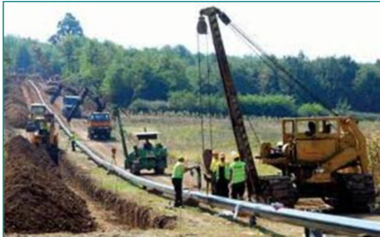
Figure 2: Construction phase of a pipeline (descent of the pipeline)
