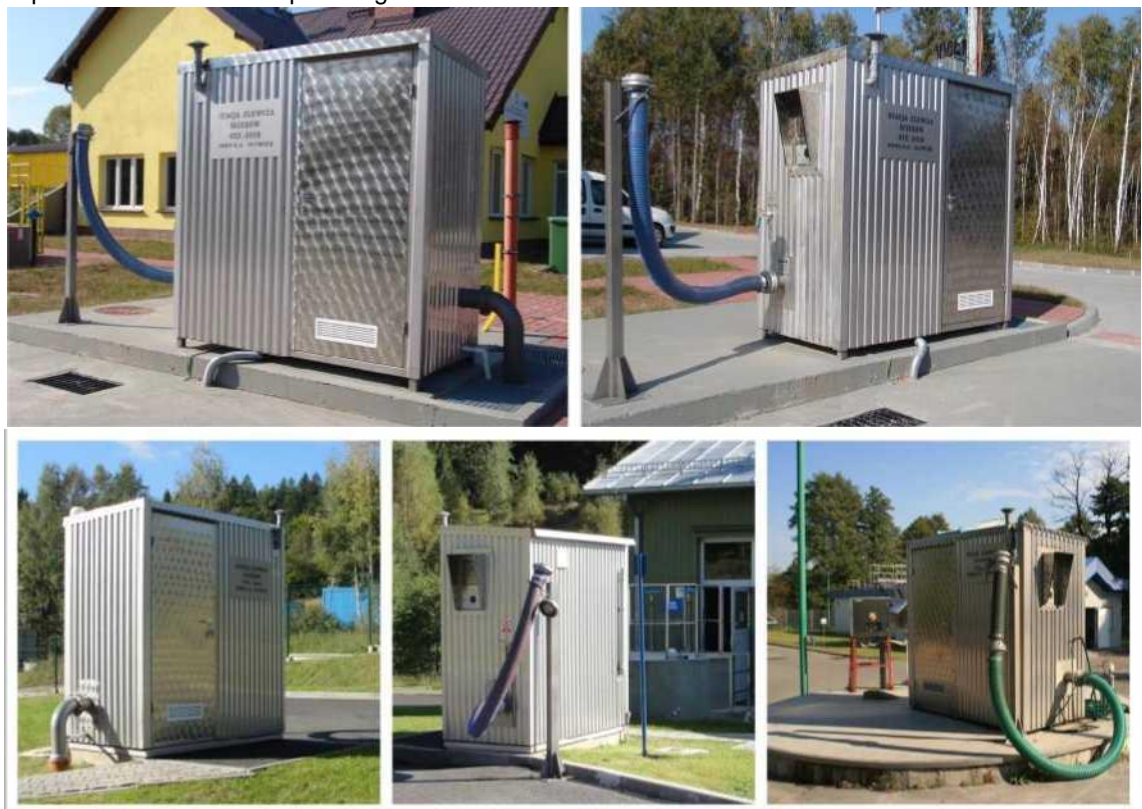
Figure 2.1 Reception node for incoming waste water
