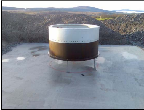
Plate 3.2 Levelled turbine tower 'can'
