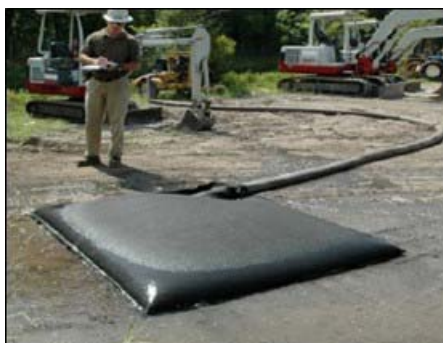
Plate 3.6 Silt Bag with water being pumped through
