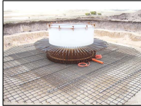
Plate 3.3 Steel reinforcement being added
