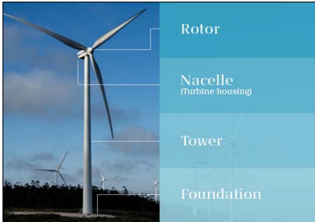
Plate 3.1 Wind turbine components
