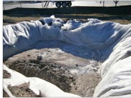
Plate 3.5 Concrete washout area
