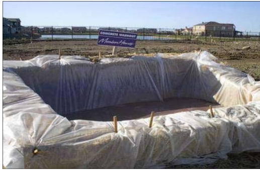
Plate 3.4 Concrete washout area
