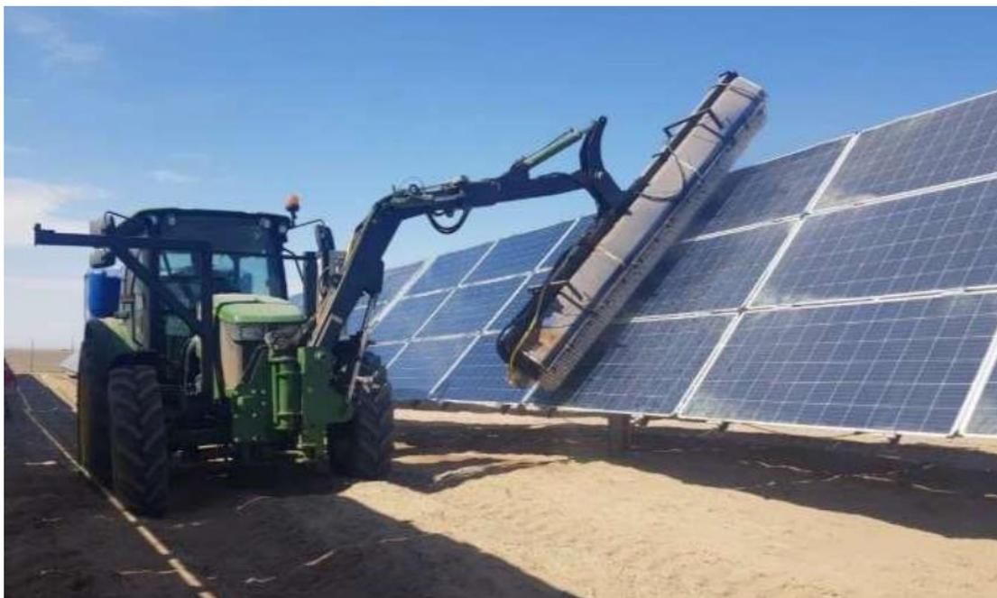
**Figure 38: Example of cleaning panels with brush**
