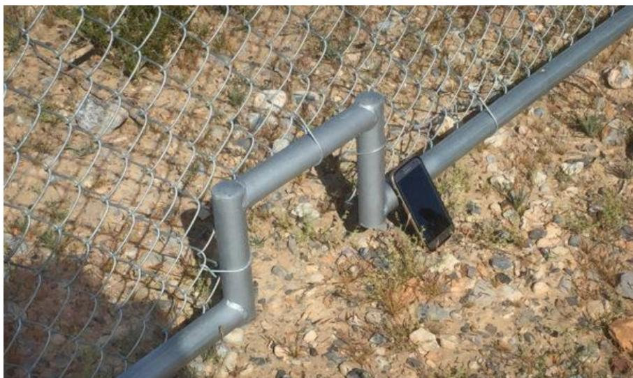
**Figure 41 Example of fence with gap for tortoises' movement and facilities for temporary storage of tortoises during operation phase**
