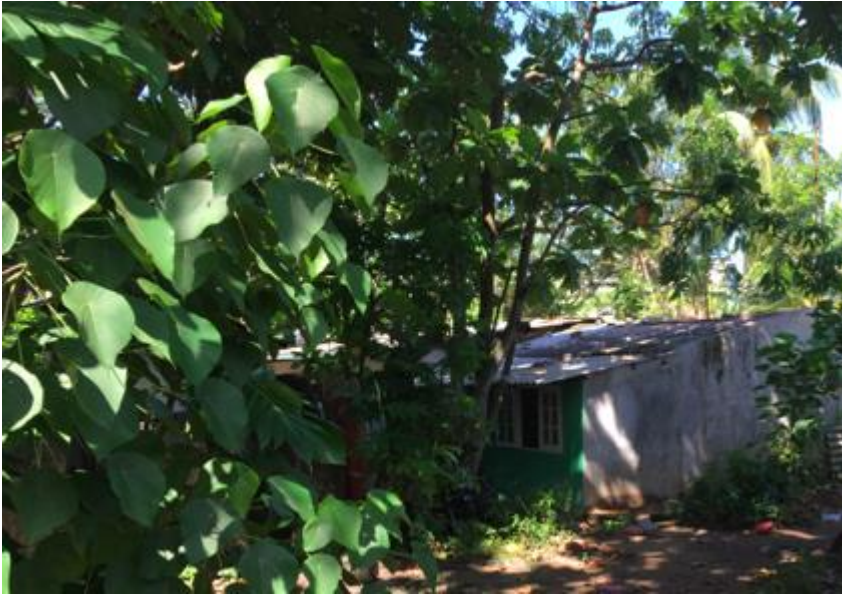
A) Pumping station 1 - "Dabare Road" pumping station
