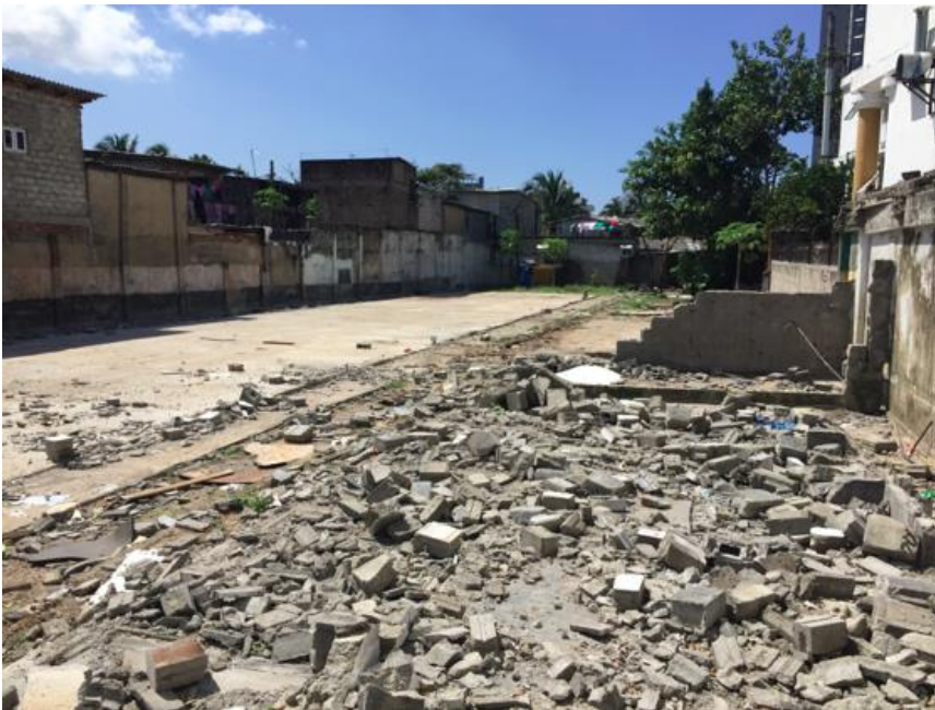
B) Pumping station 2- "Nawala Road" pumping station
