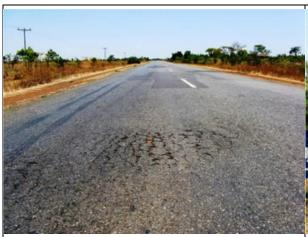
Photo 7 (km 85.2) Failing old road surface showing severe crocodile cracking and patches. Infrastructure includes telephone lines.
