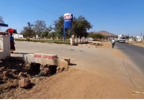
Photo 3 (km 5.3) The road surface is in fair condition but significant edge break has occurred
