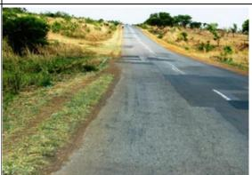
Photo 5 (km 31.4) Reconstructed gravel shoulders on a curve
