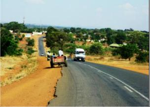
(km 132) Rumble strips lead down to a small bridge (B6). Inadequate provision for NMT on the approaches to bridge
