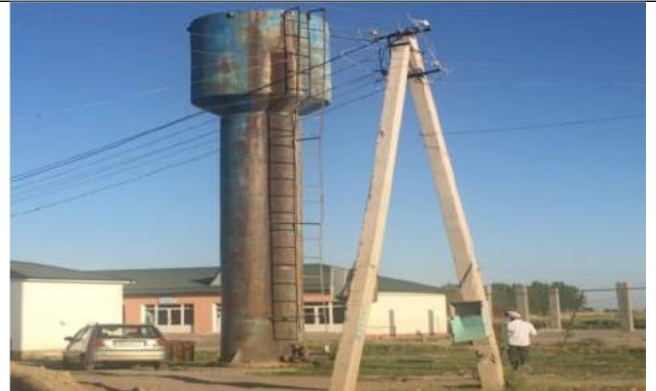
The water tower in the «Ilgor» Mahalla
