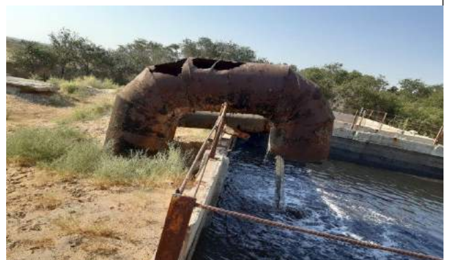
STP consist of bioproducts with several stages of purification.
