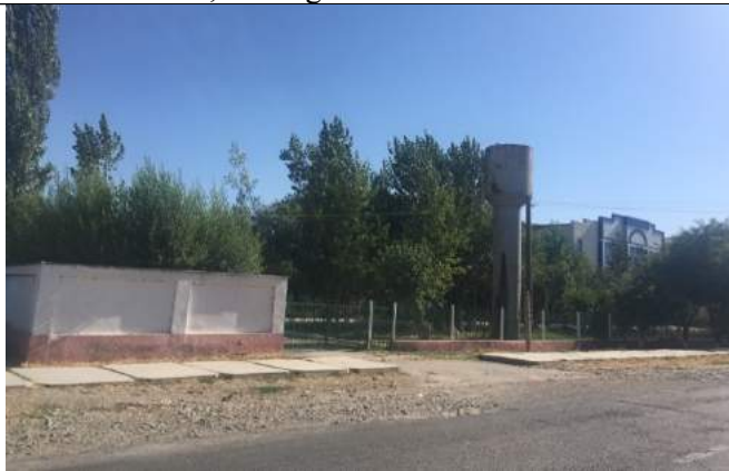
The water tower in the town of Ziyokor in Chultukai KFY.
