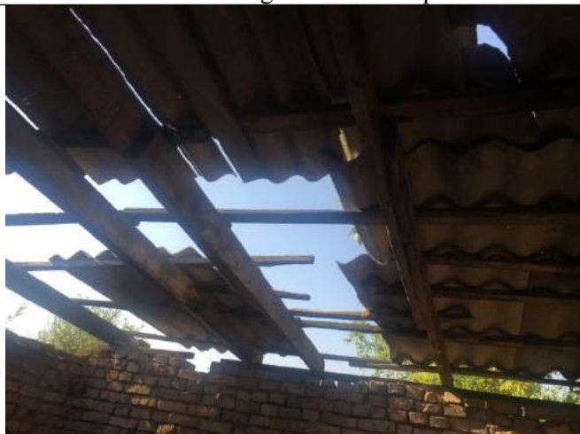
The roof of the intake structure
