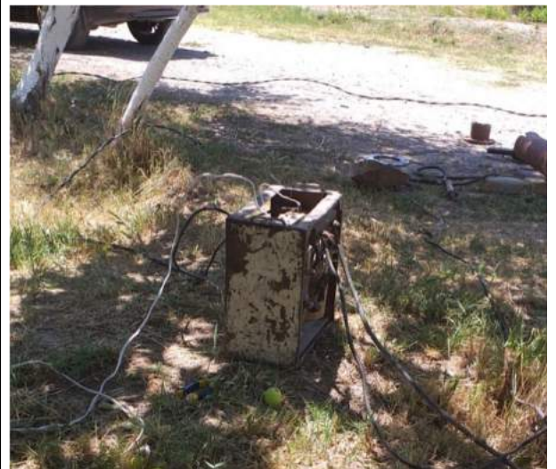
Repair works on the territory of the pumping station
