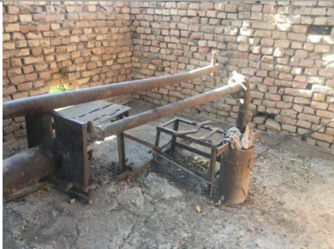
The equipment of the intake structure is severely worn
