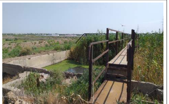
Due to the deterioration of structures, untreated wastewater is discharged to the terrain
