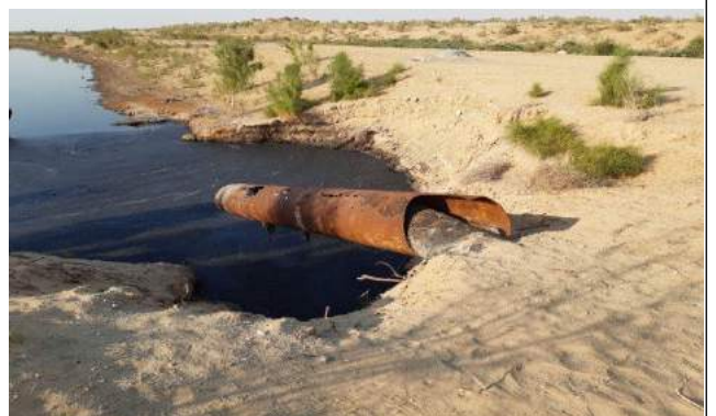
Due to the deterioration of structures, untreated wastewater is discharged to the terrain
