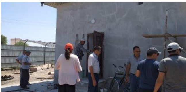
Renovated sewage pumping station in Takhiatash city
