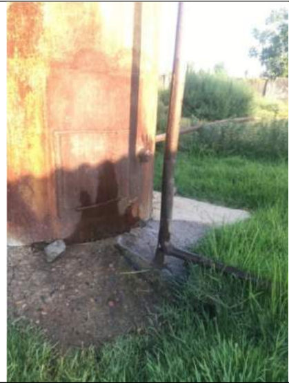
Damaged water tower body.
