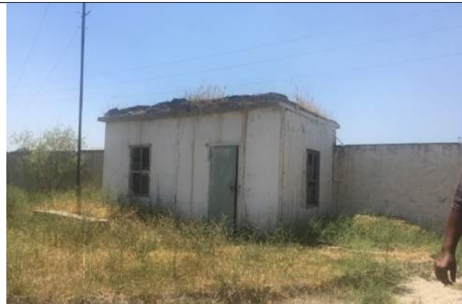
The building of water intake structures.
