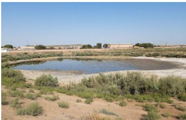
The Kungrad sewerage system was put into operation in 1970. There is no sewage treatment plant in Kungrad.
