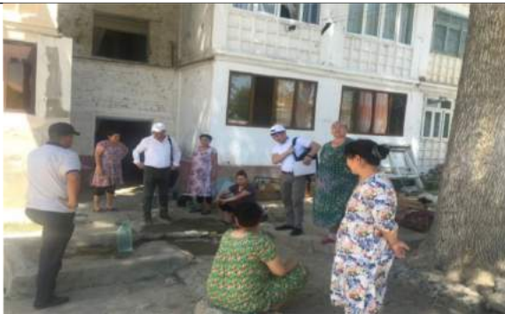
The water supply system is located in the yard of a multi-storey building. The drinking water pipe has been damaged. Water is mixed with sewage and is not suitable for drinking.
