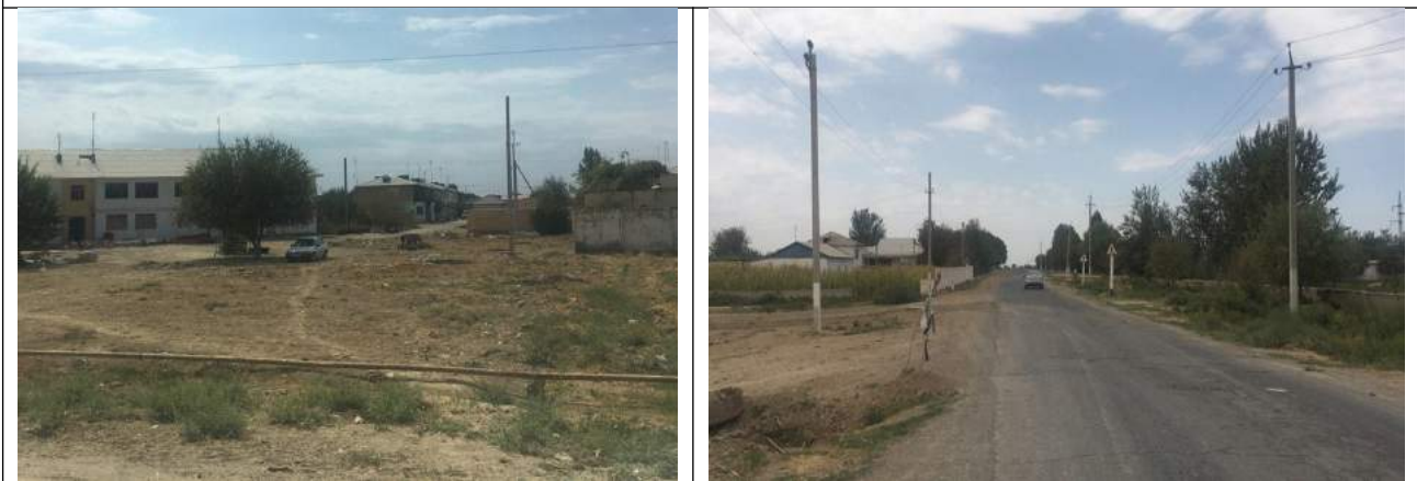
A fragment of the street where the sewerage network and gravity flow collector will pass
