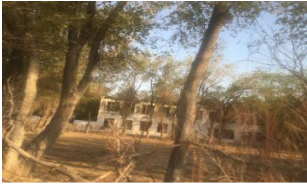
Building of the main sewage pumping station
