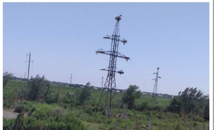
Red Listed storks nesting on high-voltage lines near the STP.
