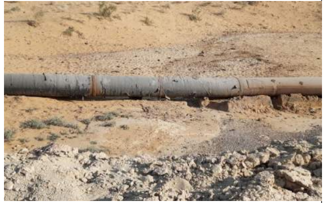
Wastewaters from the sewage treatment plant are directed through the pipeline to the filtration fields located in Kyzylkum
