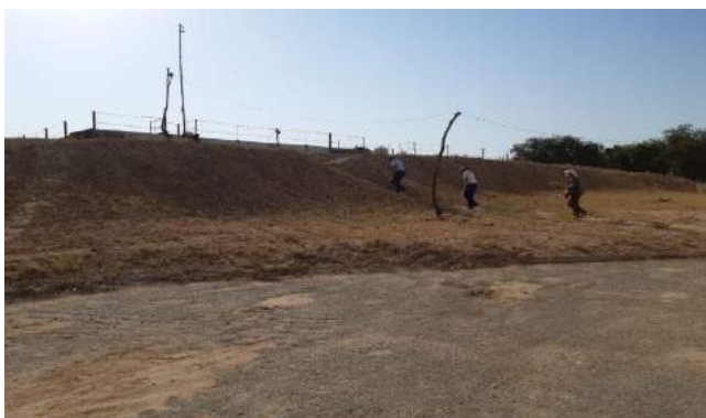
STP in Nukus was put into operation in 1984. Design capacity was 65 thousand m 3 /day.
