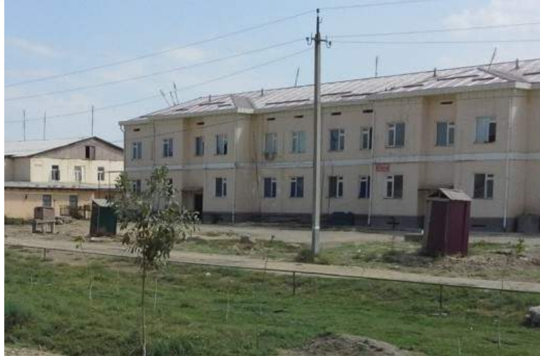
In the foreground of the photo there are individual toilets (cesspools) built by the residents of a two-storey residential building.
