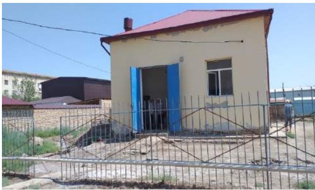
Private sewage pumping station, transferred to private use in the city of Takhiatash. Serves multi-storey buildings located nearby
