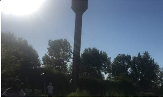
Water Tower in Mahalla "Intilish". From the body of the water tower, water gushes forth.
