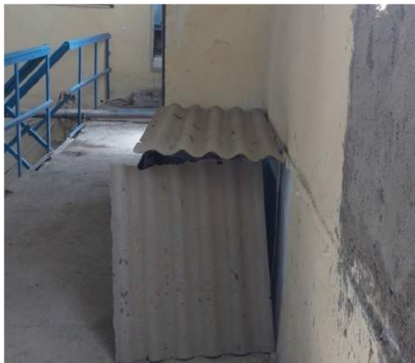
Asbestos sheets used as a fence
