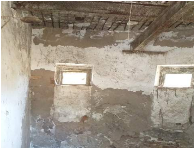
Internal view of the sewage pumping station building
