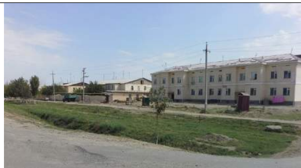
Pakhtaabad District Centre, a street to be canalized
