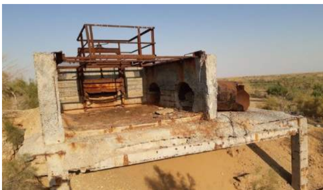
Wastewater distribution facility
