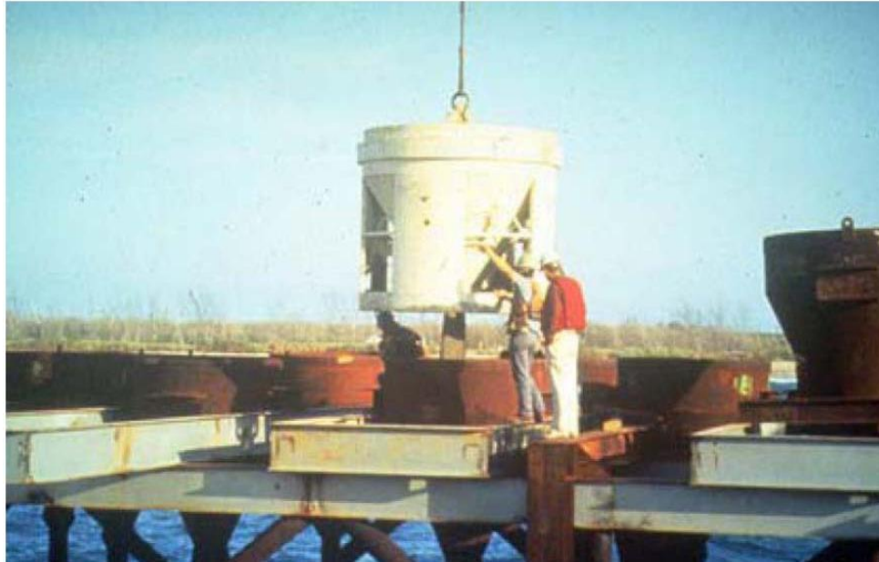
Plate 42: Conventional concrete placement using a tremie
