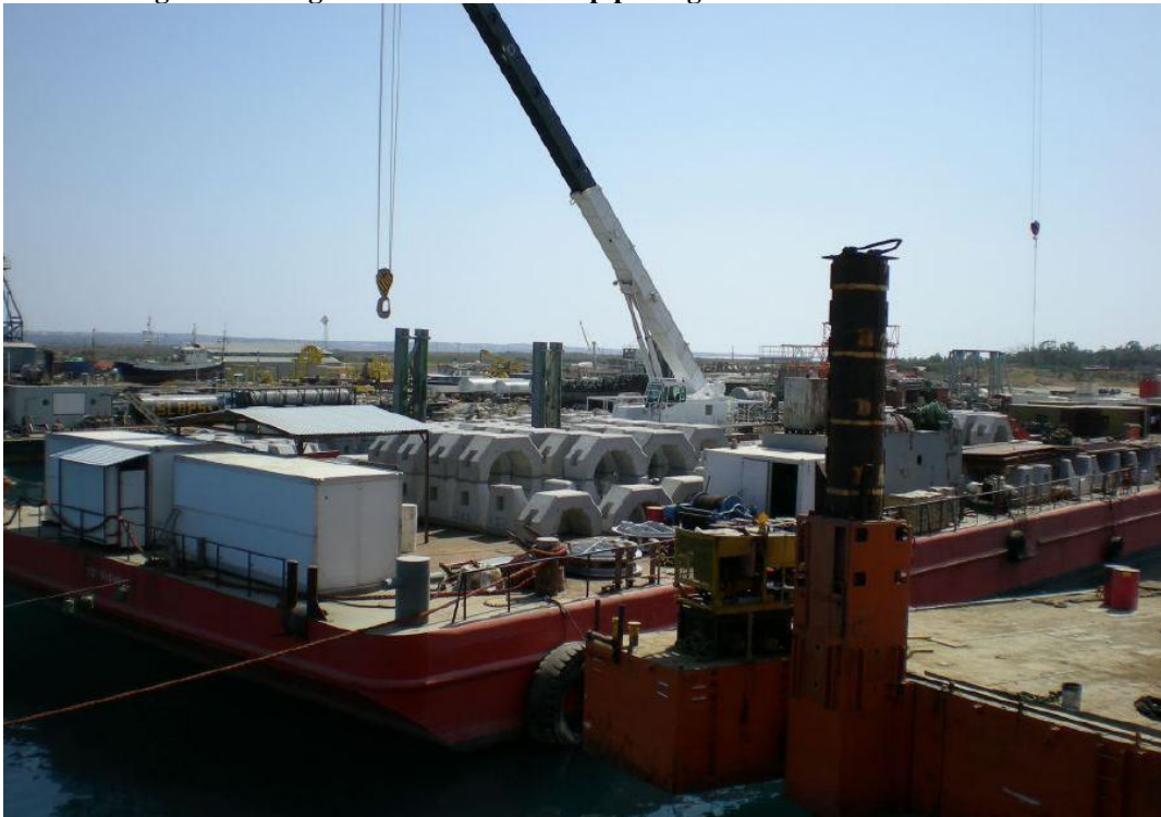
Plate 47: Precast ballast manufactured ahead of time and loaded on a barge
