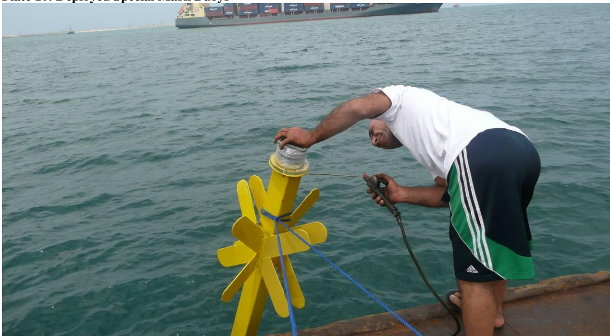
Plate 11: Welding the screws holding the lights on Buoys B-3
