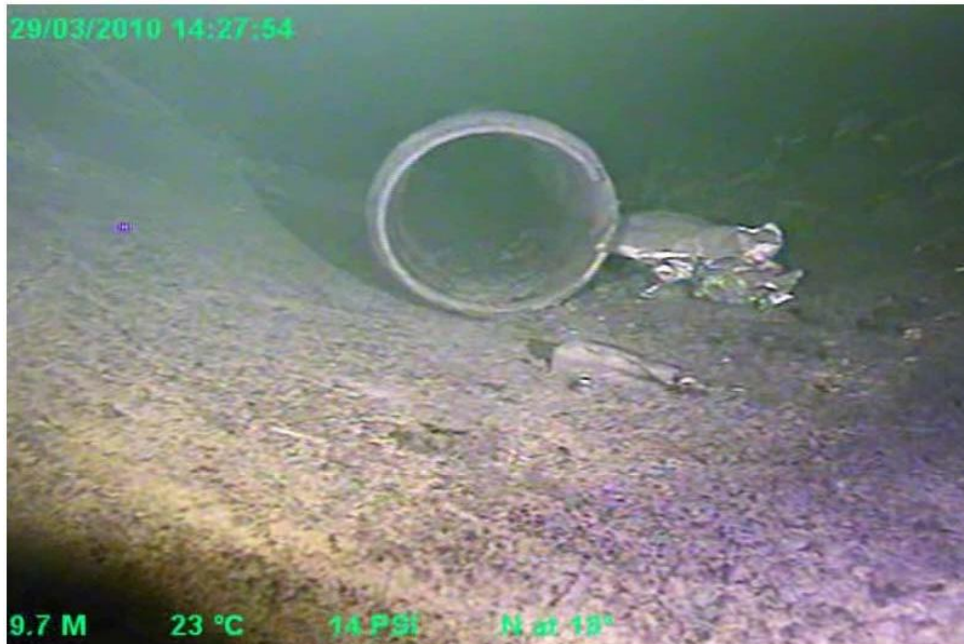
Plate 21: Debris inside the Overflow Pipe
