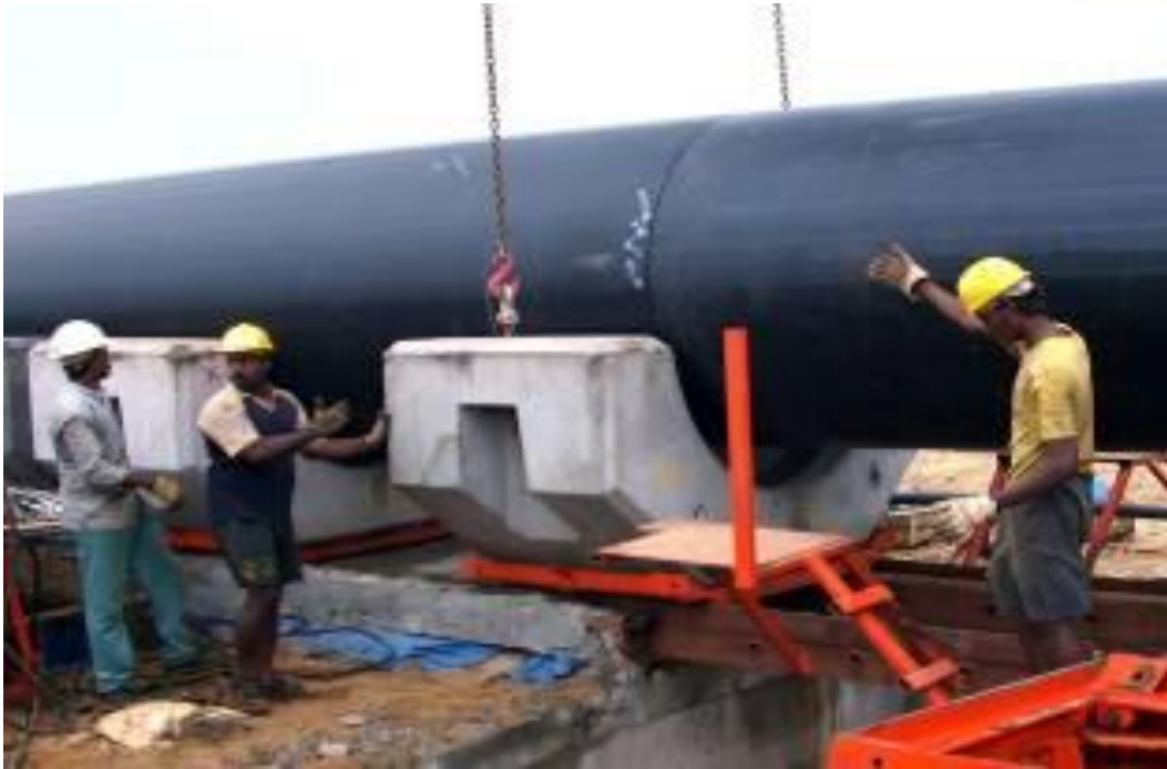
Plate 50: Butt fusion welds of pipe sections
