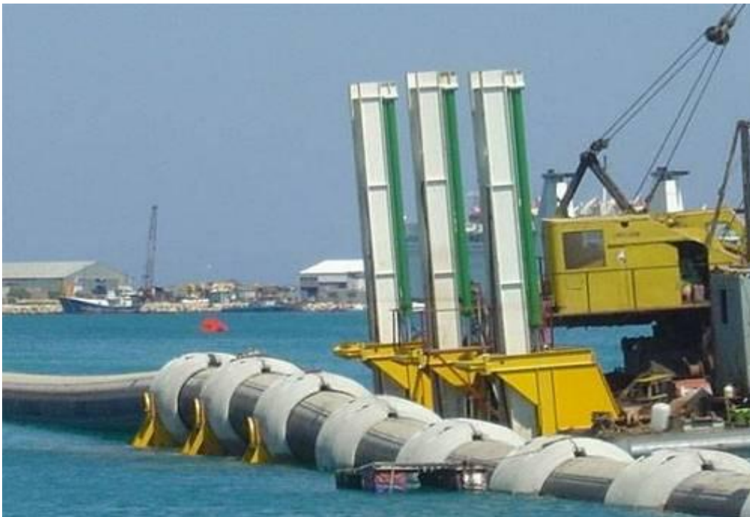
Plate 51: Installing precast ballast blocks
