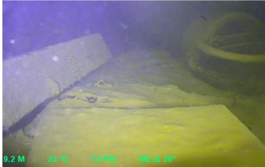
Plate 20: Large debris inside the Outfall Pipe
