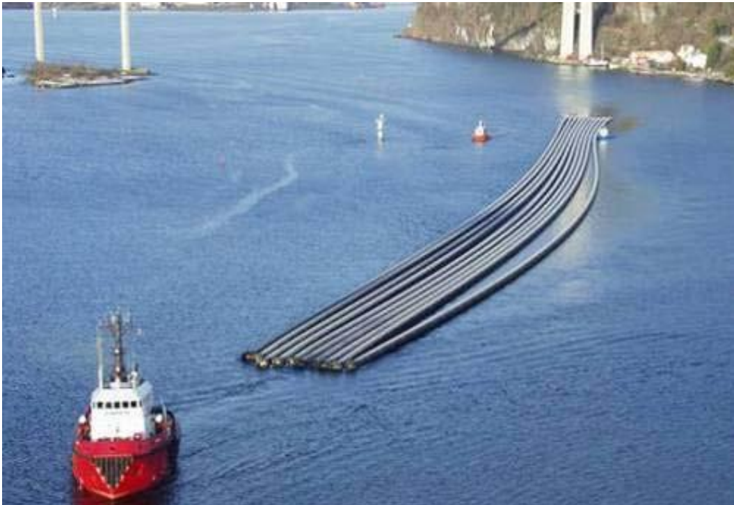
Plate 46: Tug boat towing 10 sections of HDPE pipe lengths
