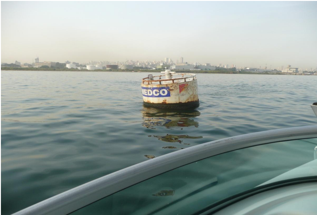
Plate 3: Steel cylindrical buoy used by tankers for off loading fuel
