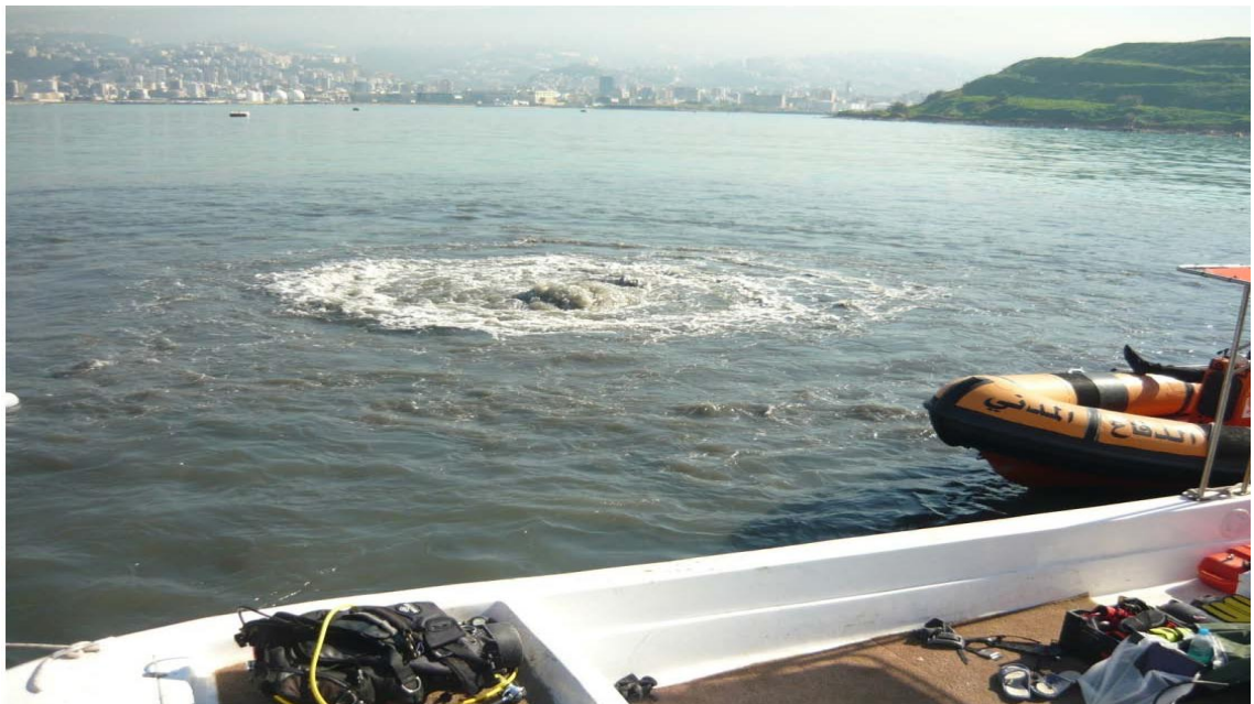
Plate 18: Dredging by air lifting techniques on-going
