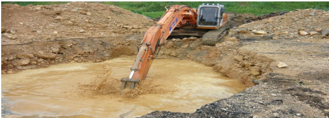
Plate 14: Excavation of trial pits on land
