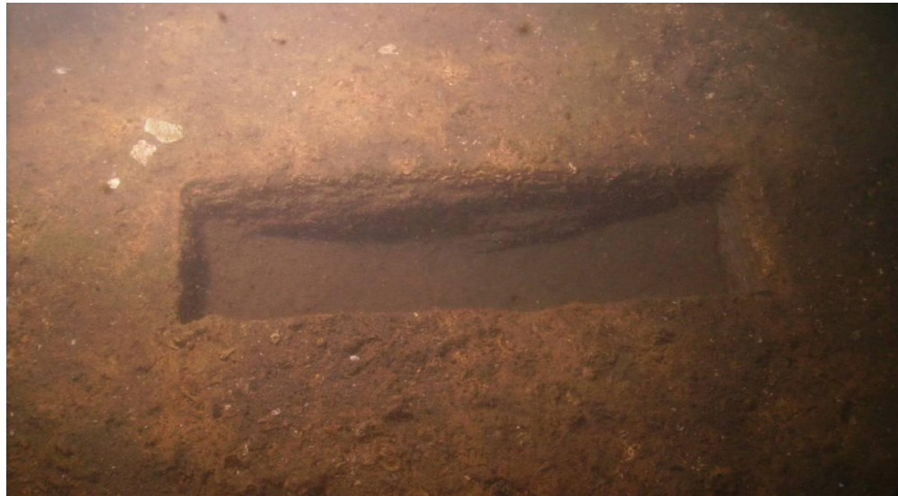
Plate 25: Typical sacrificial anode in the concrete coating of the Overflow Pipe now partially filled with silts
