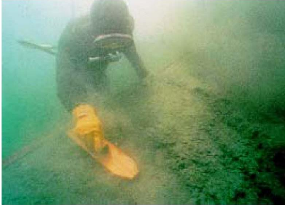
Plate 44: Concrete finishing underwater
