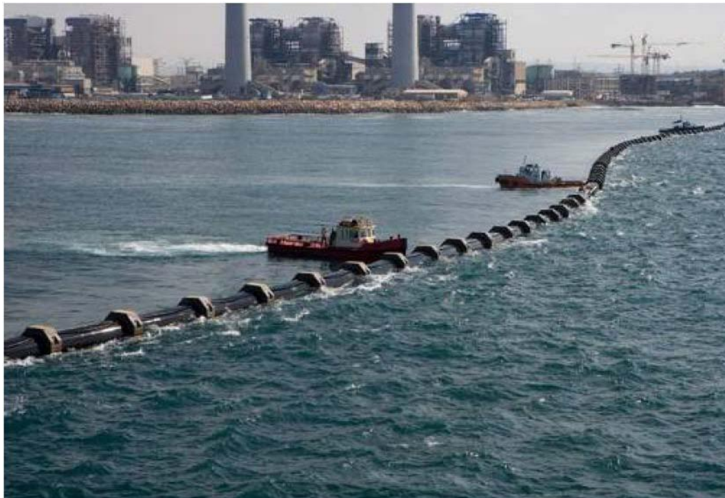
Plate 53: Aligning the pipe as required
