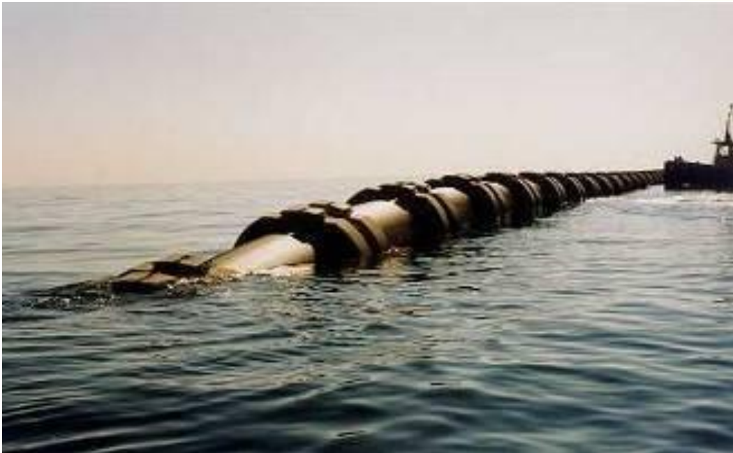
Plate 54: Flooding the pipe and sinking it
