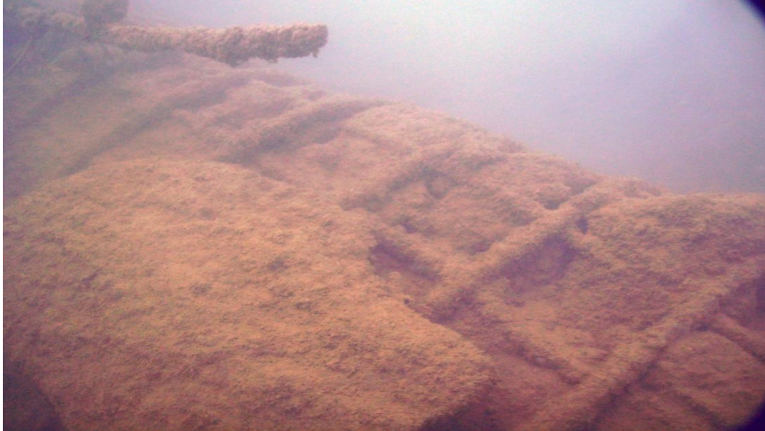
Plate 15: Exposed damaged reinforcement bars following dredging activities
