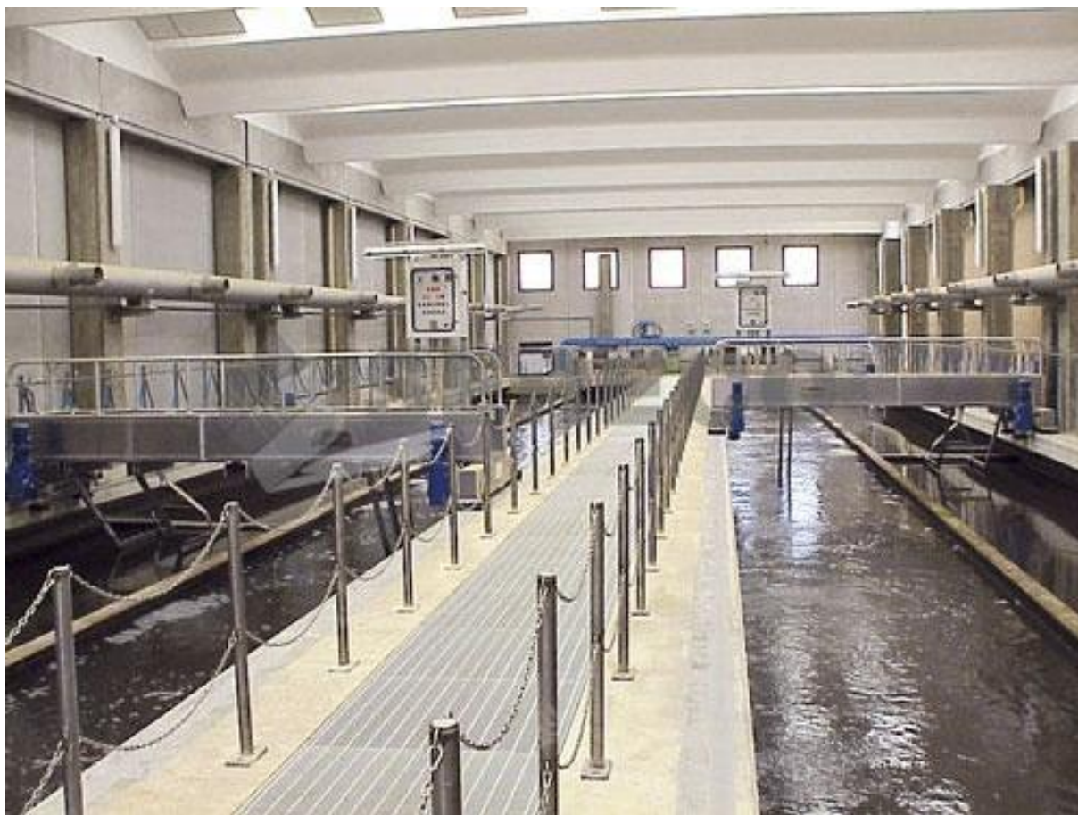
Figure 3: Aerated Grit Chambers inside an enclosed building
