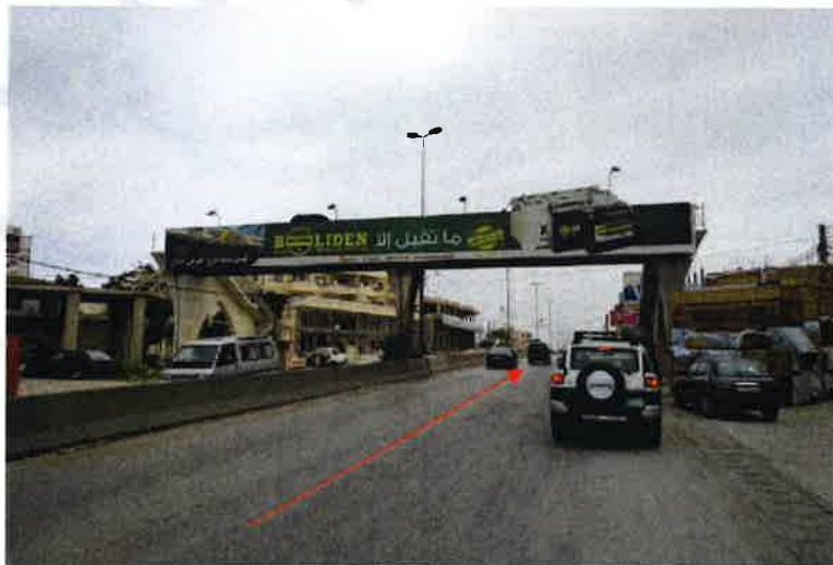
PP22. Underpass Tunnel Grid N 34.49882, E 35.960169 To the right there is a slip road off and back onto the main highway. This bypass road has no overhead restrictions and is suitable for all WTG OOG components to pass.
