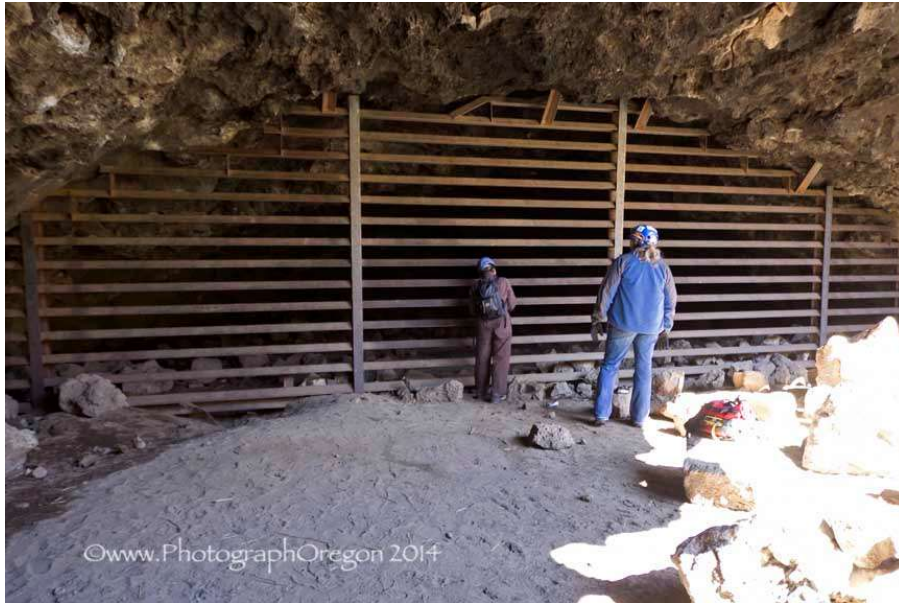
Plate 12. Photo taken from the web 1 for an example of a cave gate
