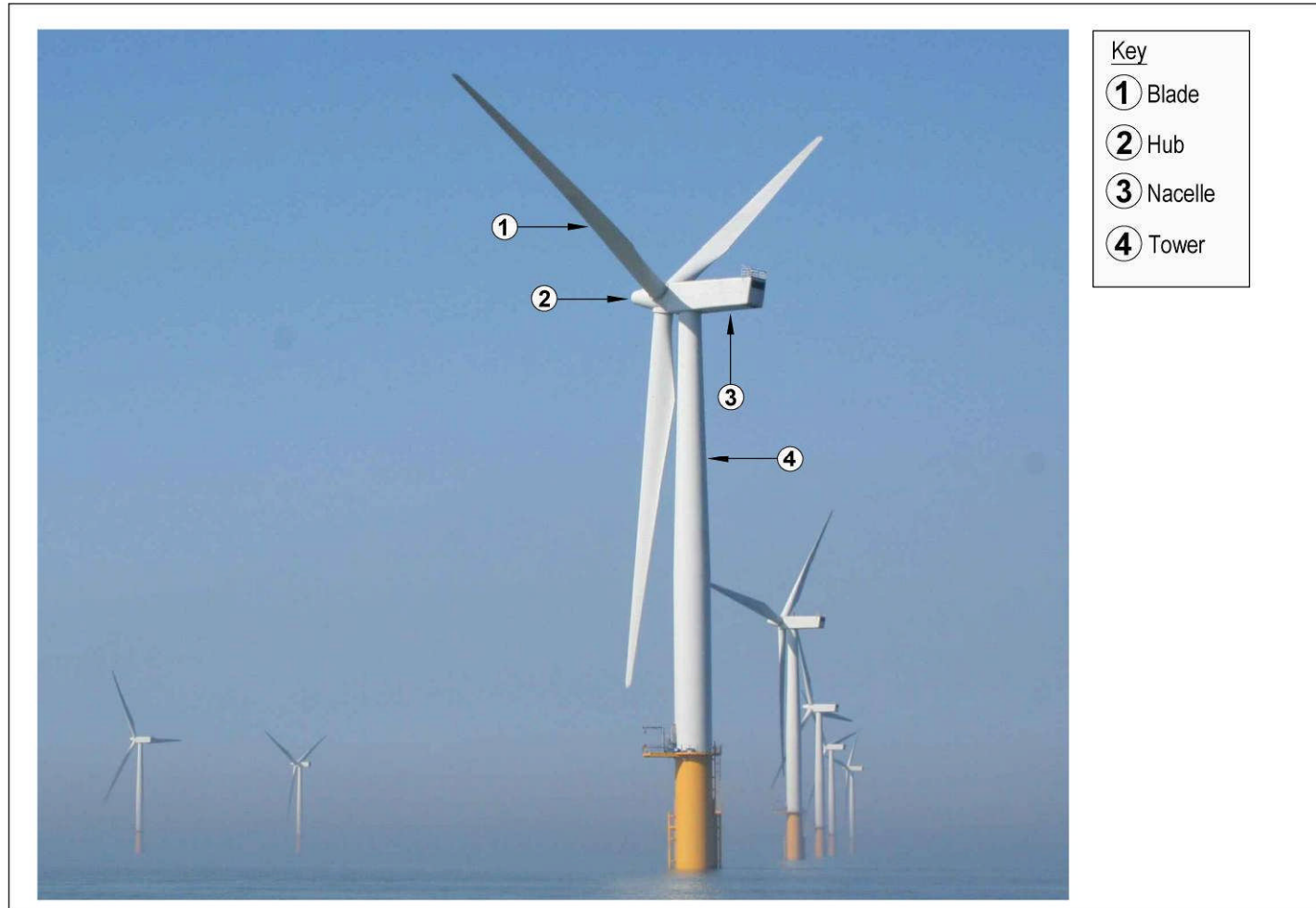
Figure C: Main wind turbine components
