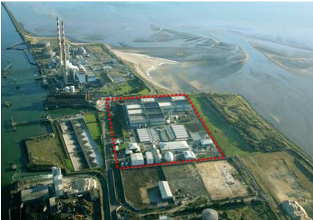
Figure 1 Aerial View of Ringsend WwTW
