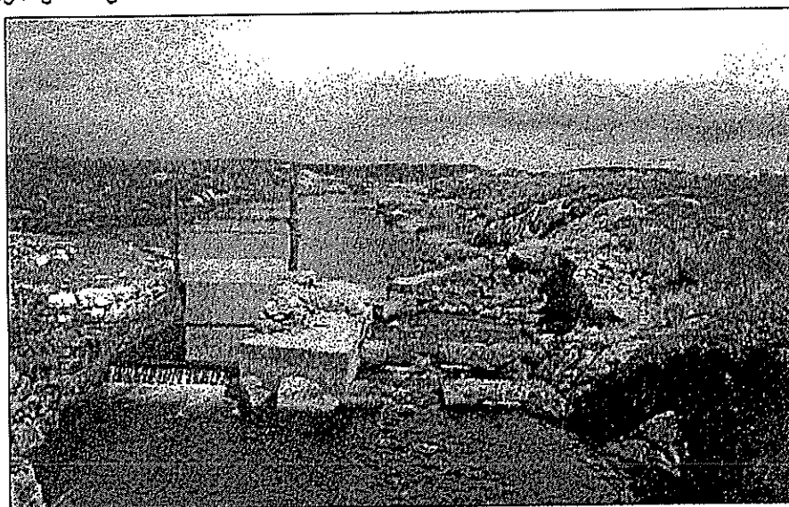
Plate 3.1 Glenicmurrin Lake Outlet Control Structure – looking upstream
