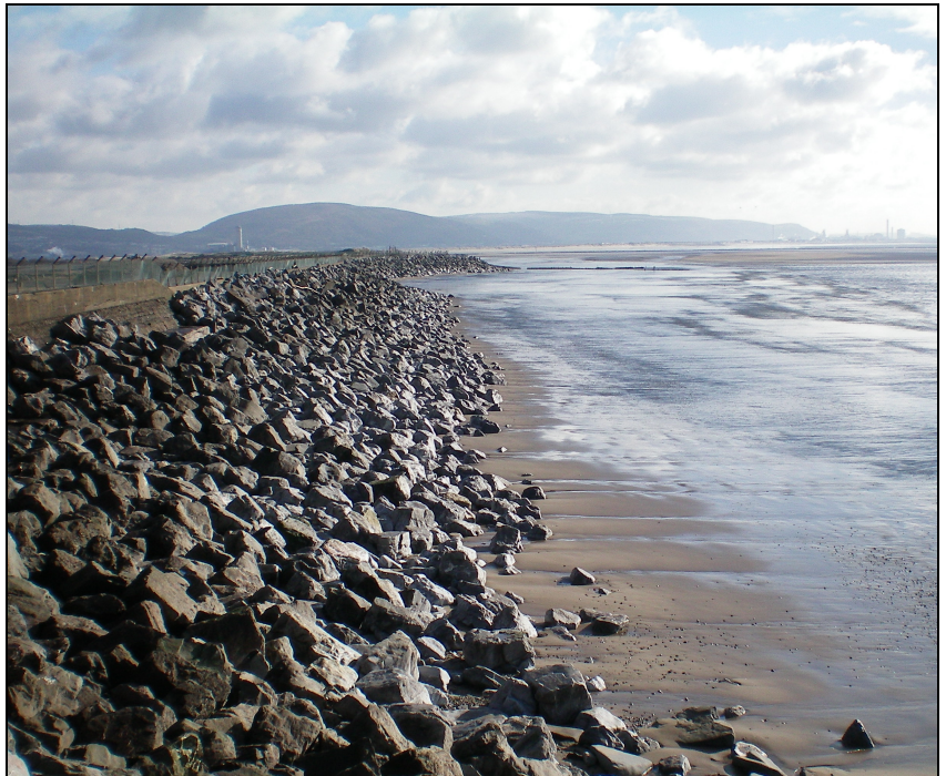
Figure 7: Existing Rock Revetment within the Proposed Development Site Boundary
