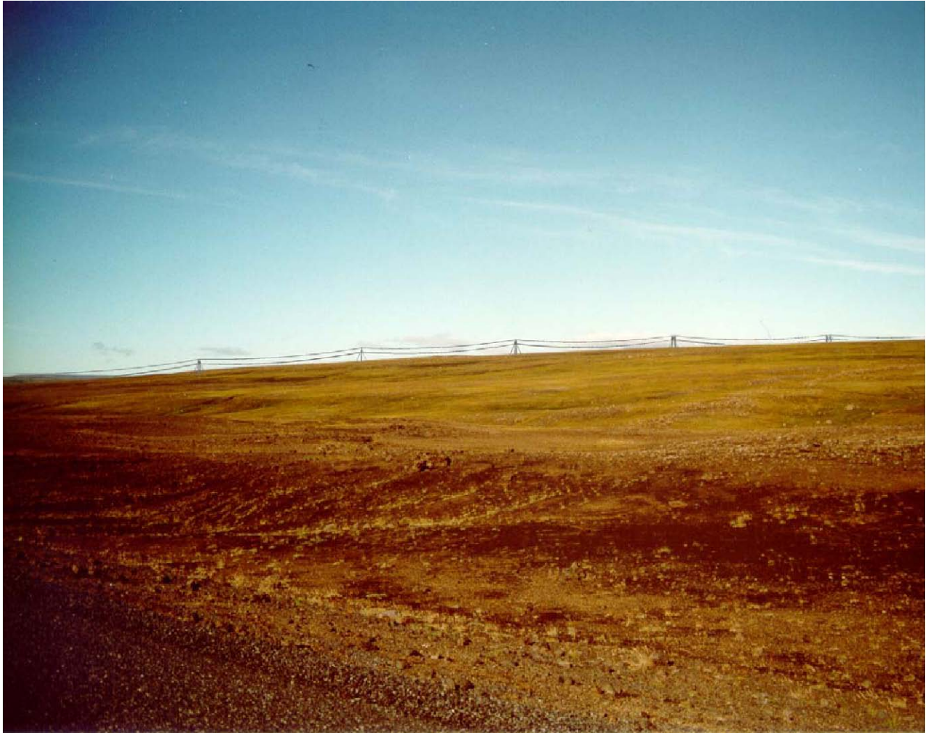
Fig. 5.7 Búðarháls line 1, looking northwest over Búðarháls from Highway 26. Both the towers and the wires are indicated more clearly by having them a darker colour than they will actually be.
