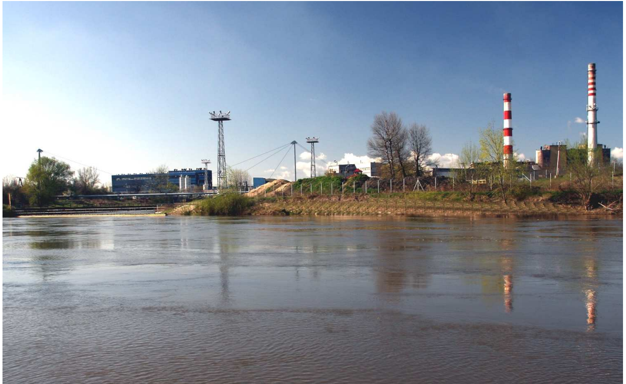
Photo 3. Location of the planned waterside pumping station to be erected in the San River's bay.
