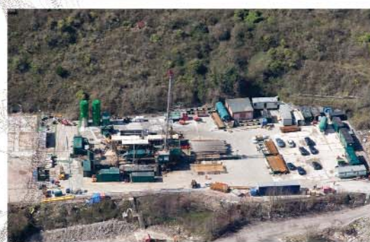
Drilling of well Portland - 1/1A in 2006
