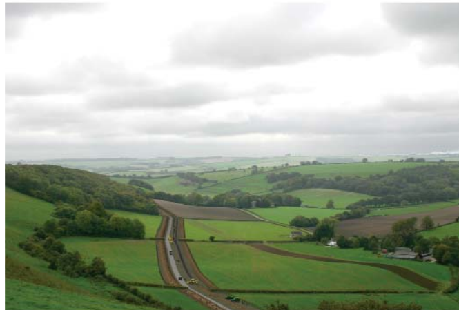
Lyscombe Hill in construction
