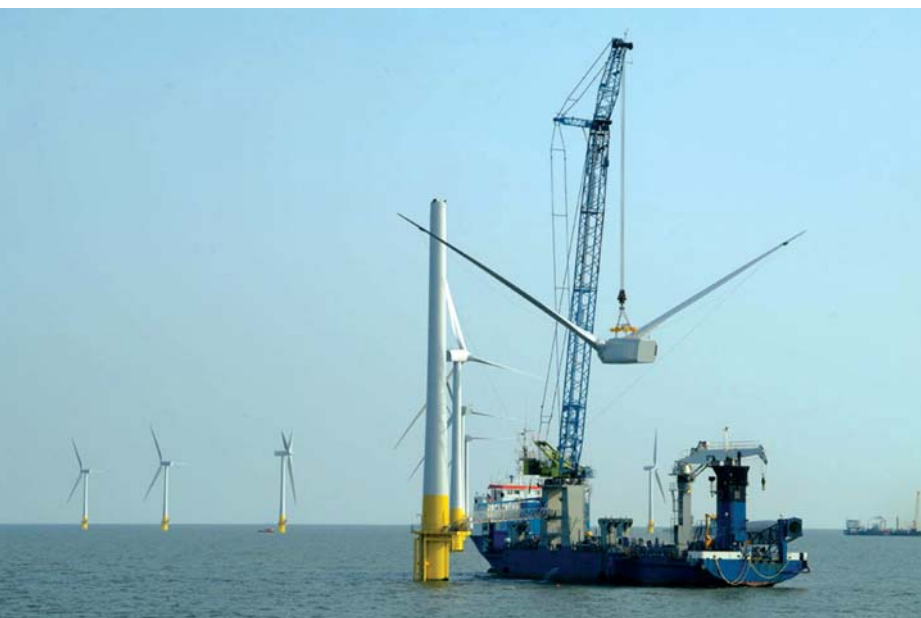
Installation of an offshore wind farm
