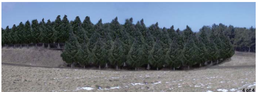
Figure 4 - Photomontage of proposed landscaping shielding new Switch Room at The Muckleburgh Collection, Weybourne, Norfolk.
