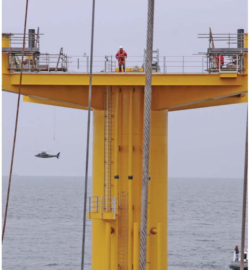
Installation of offshore substation (Barrow, 2006)
