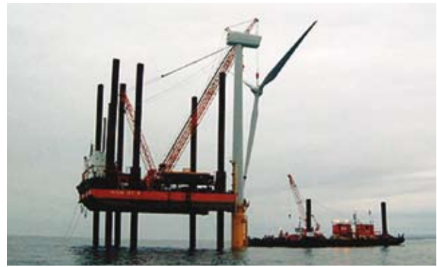
Figure 3: A Jack-Up Installation Rig with Attendant Barge (Source: Seacore)
