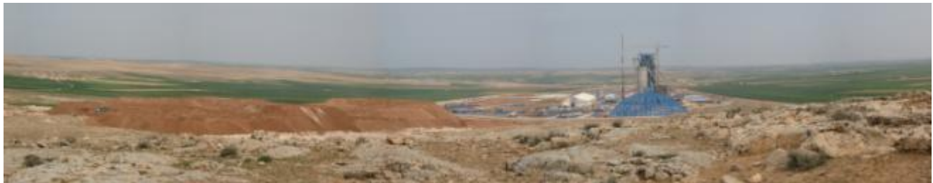
Figure 6-1 View of Plant Site (130ha) from Jabal Koujak
