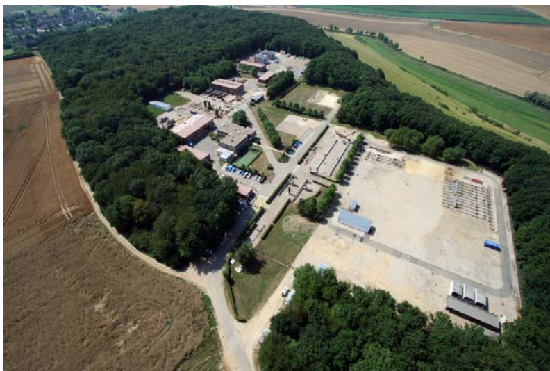
Figure 1 : La station centrale.
