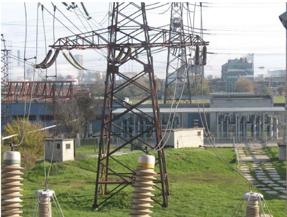
Figure 5. The switching port of pressure conduits
