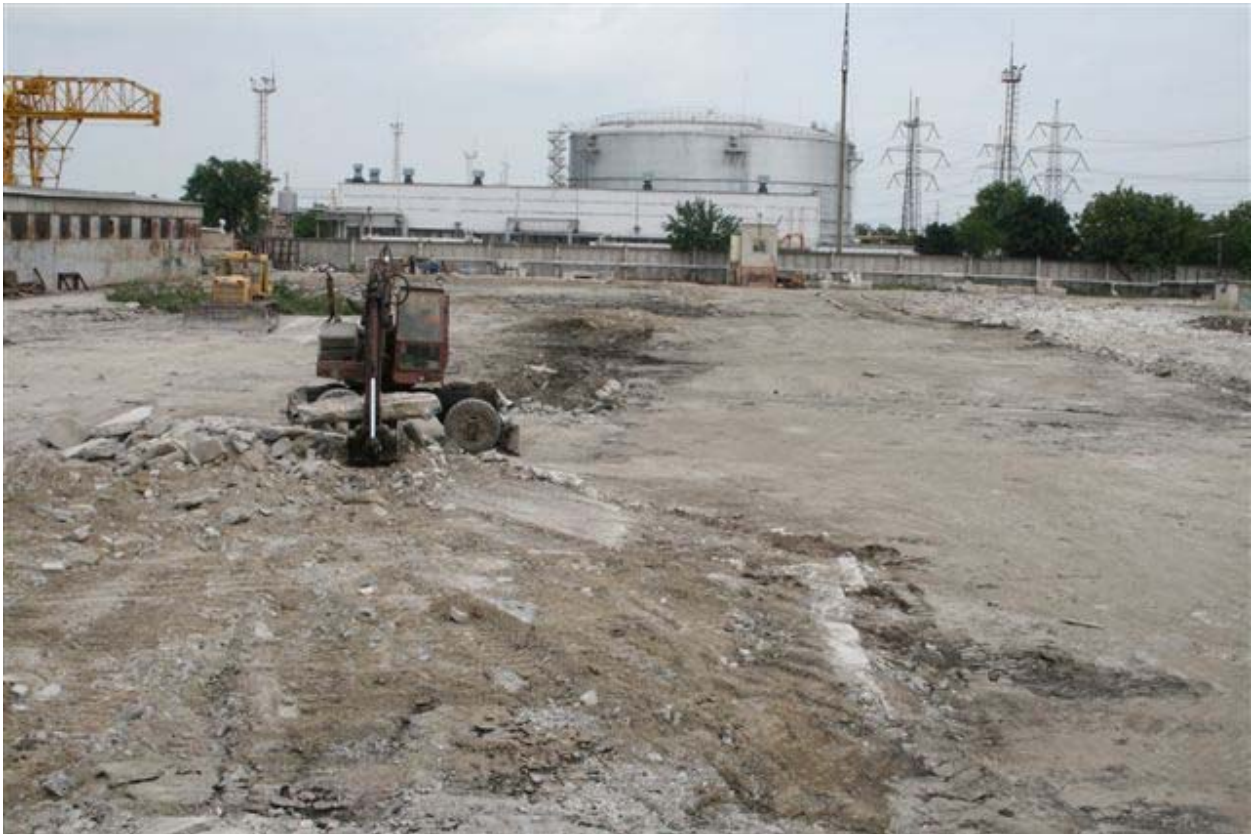
Figure 3. The existing condition of the site for the construction of CCGT-410
