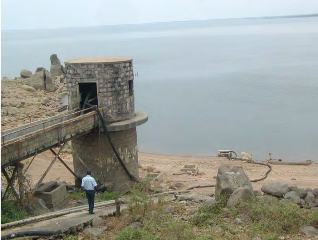
Figure 9: Water pumping station for the water treatment plant at Itezhi-tezhi
