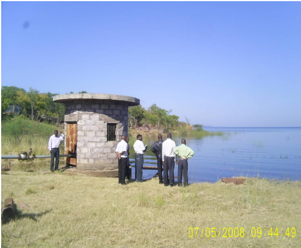
Figure 21 Water pumping station for the water treatment plant at Itezhi-tezhi
