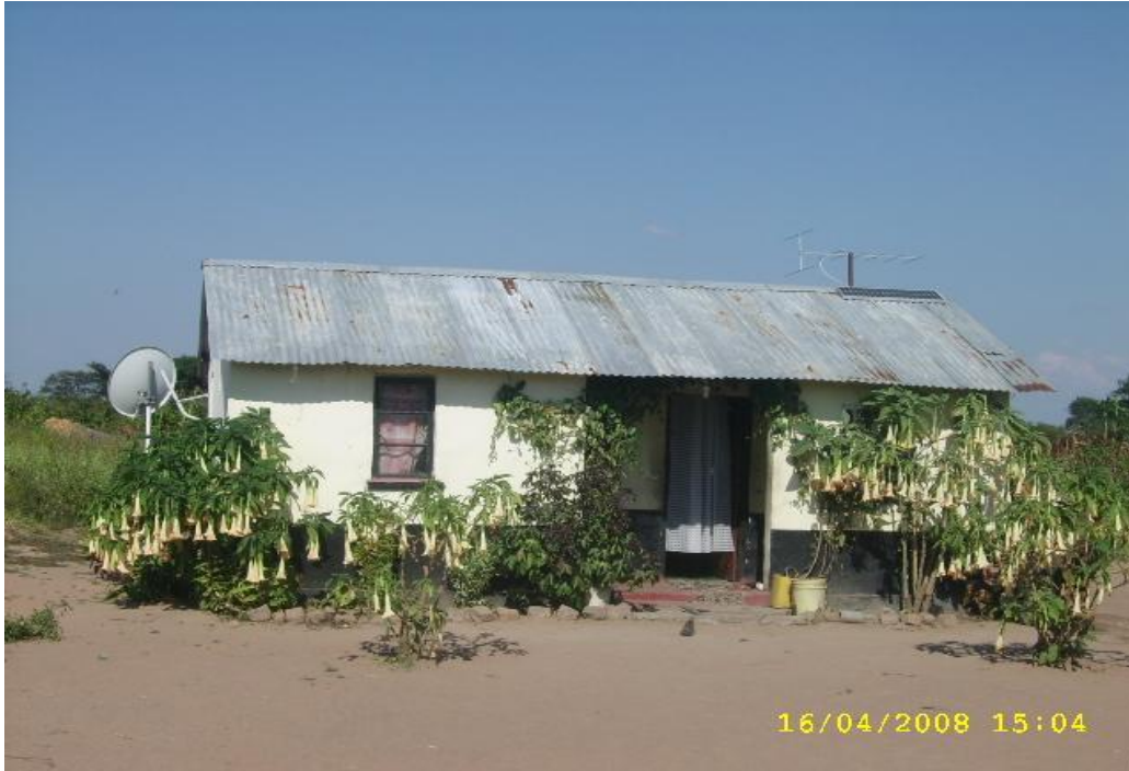
Figure 16 Improved dwelling structure in Lubanda Village.
