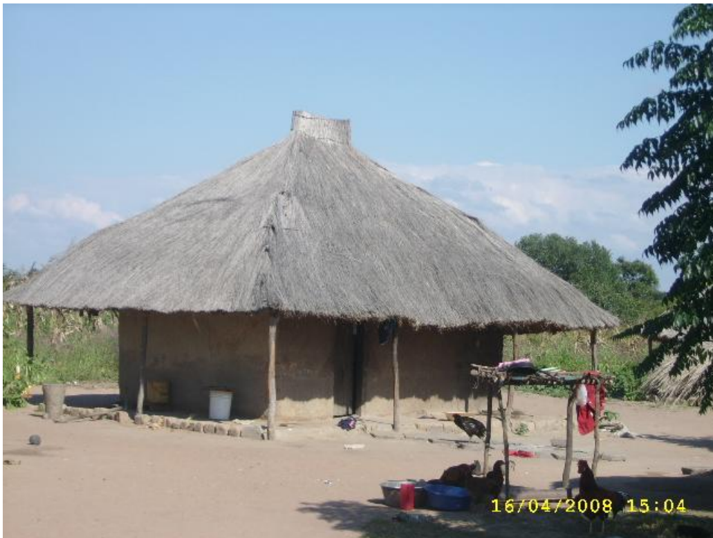
Figure 15 Typical common dwelling structure in project area (Lubanda)
