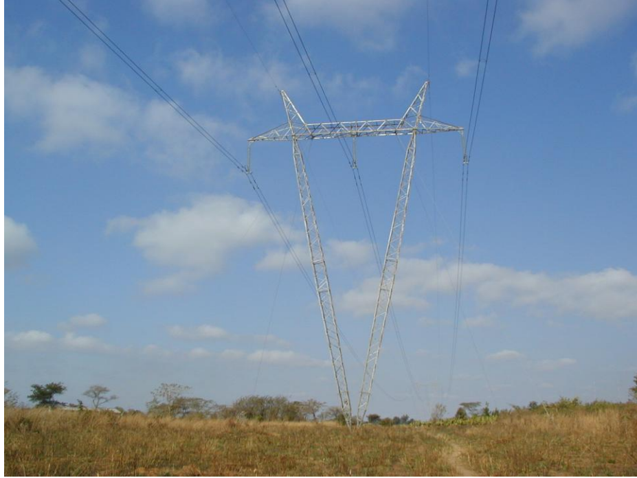
Figure 3 Guyed Vee 330kV tower structure
