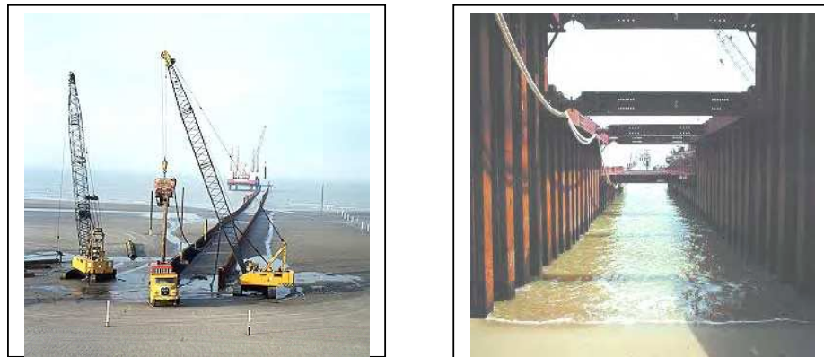
Figure 3.10 Illustration of a Typical Cofferdam Construction
