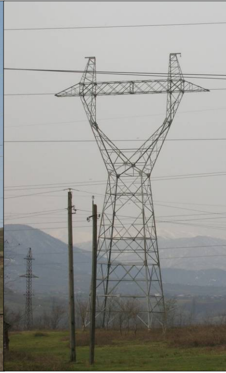
Single 4-point contact steel lattice tower. Used primarily for in-line conductors
