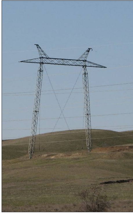
H-Frame 2-point contact steel lattice tower. Used primarily for in-line conductors.
