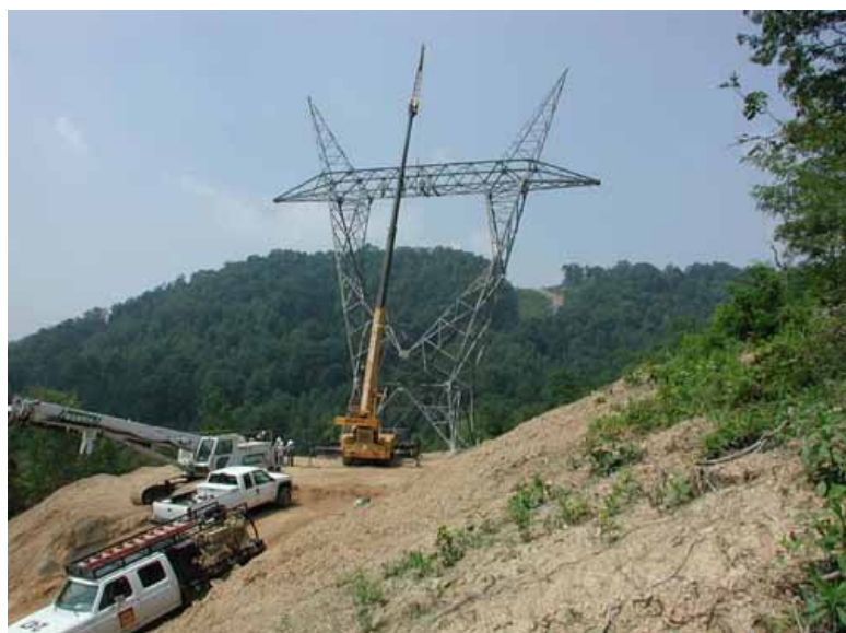
Figure 2-4. Raising tower in mountainous terrain
