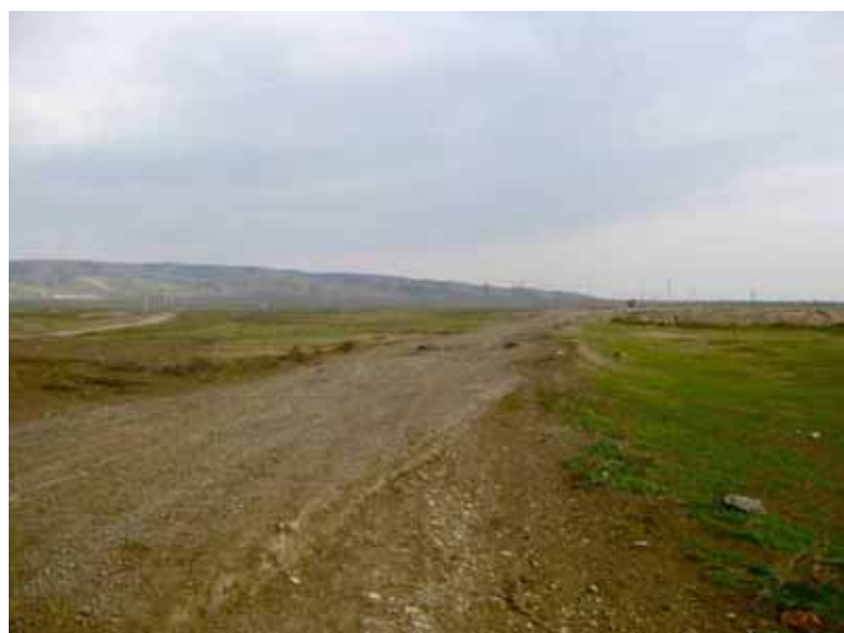
Figure 4.2-2. Typical secondary road along the transmission line route. Original paved route has been abandoned for successive unpaved tracks.
