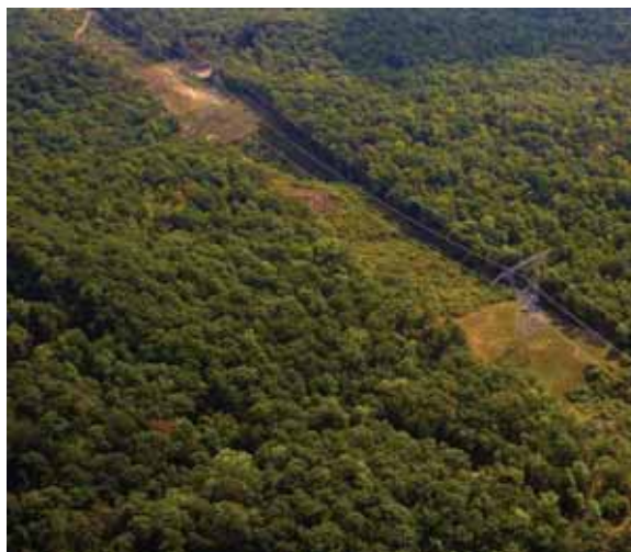
Figure 2-7. Example of vegetation clearing for corridor maintenance in forested terrain
