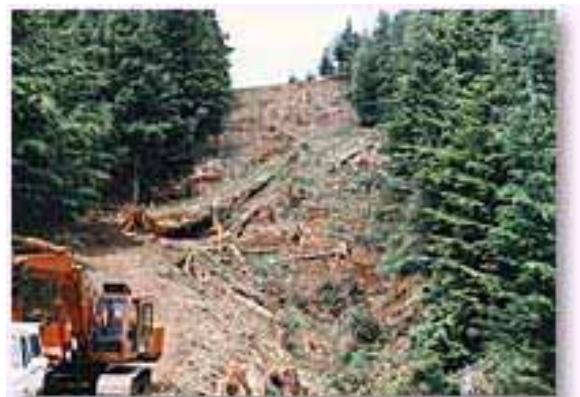
Figure 2-2. Vegetation clearing of a narrow corridor
