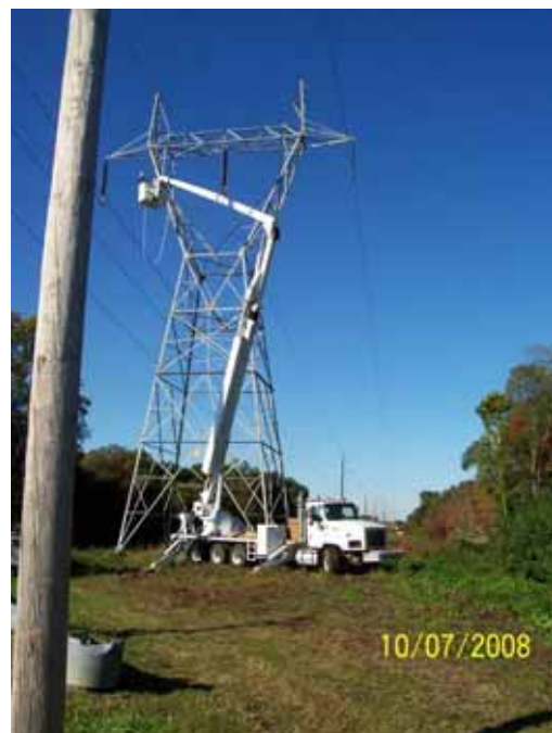
Figure 2-6. Ground-based conductoring
