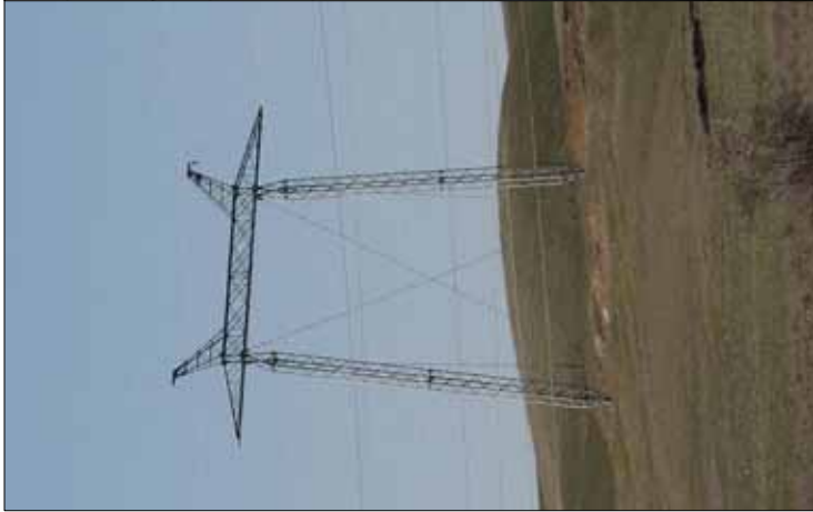
H-Frame 2-point contact steel lattice tower. Used primarily for in-line conductors.
