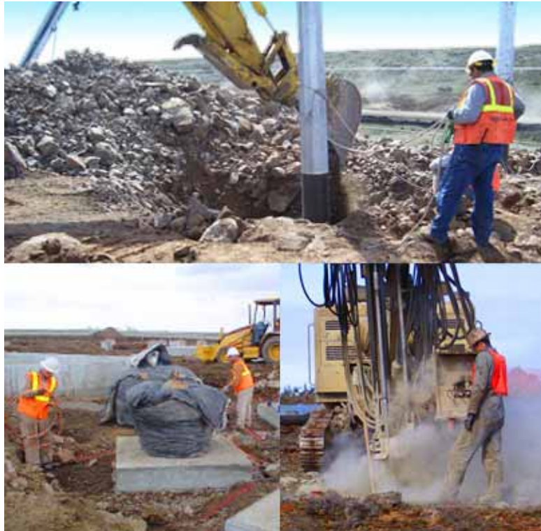
Figure 2-3. Typical installation of foundations and setting towers
