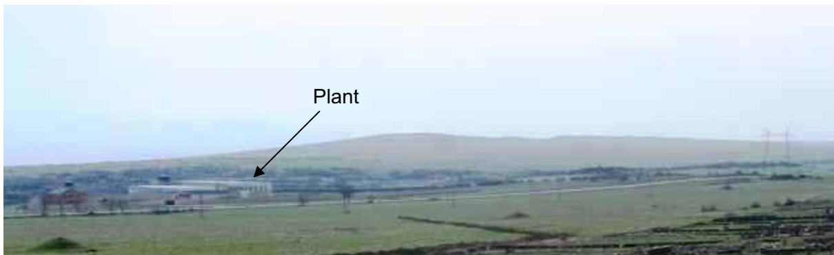
Figure 4.2-5. Basalt processing plant near proposed transmission line (plant is at left center, tower for proposed line visible at right)
