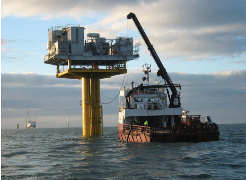
Installation of offshore substation
