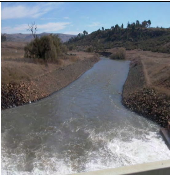
Photo 19: Downstream view from Boston A Dam.
