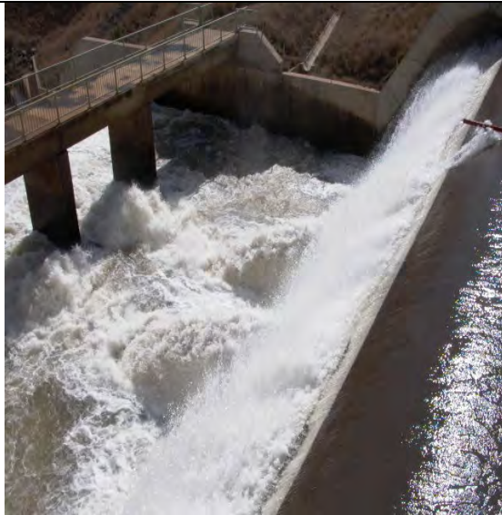
Photo 23: Water outlets at weir indicating proposed location of penstock connections.
