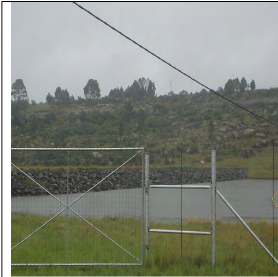
Photo 9: Use of granite rock and gabions for construction of a weir which in turn also prevents sedimentation load and erosion.
