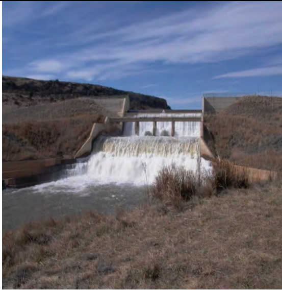
Photo 17: The proposed site for establishment of the Hydro Power Plant.
