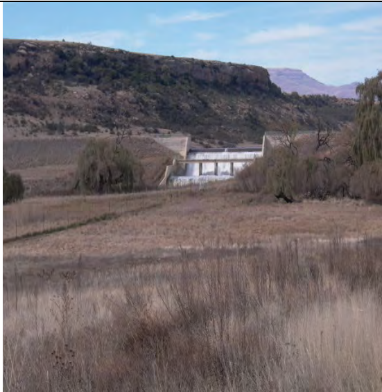
Photo 27: View of Boston A Dam weir from adjacent farm.
