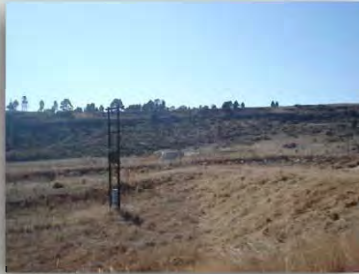
CURRENT VIEW TOWARDS EXISTING DAM WALL STANDING ON THE DE KRANS DAM WALL
