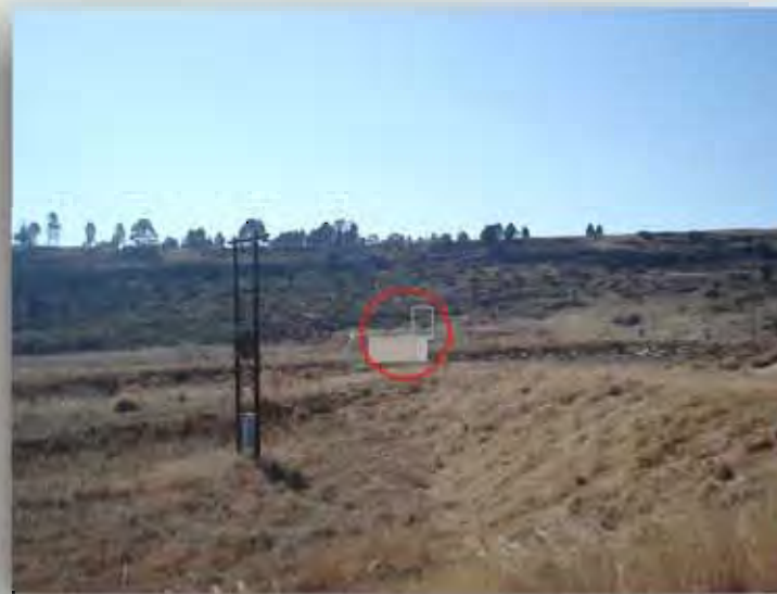
VIEW TOWARDS EXISTING DAM WALL WITH HYDRO IN POSITION STANDING ON THE DE KRANS DAM WALL
