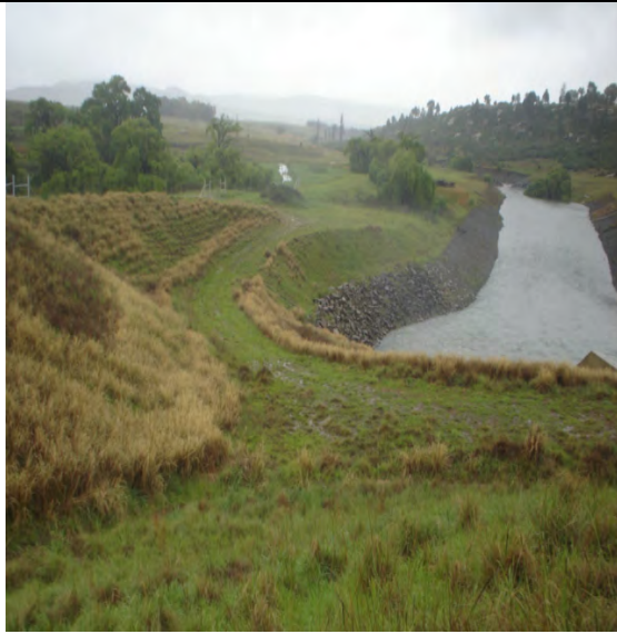
Photo 1: View of the proposed site for the construction of the Hydro Power Plant (south west of the Boston A Dam).
