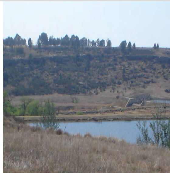
Photo 16: View of the private dam as well as Boston A Dam from an adjacent farm.
