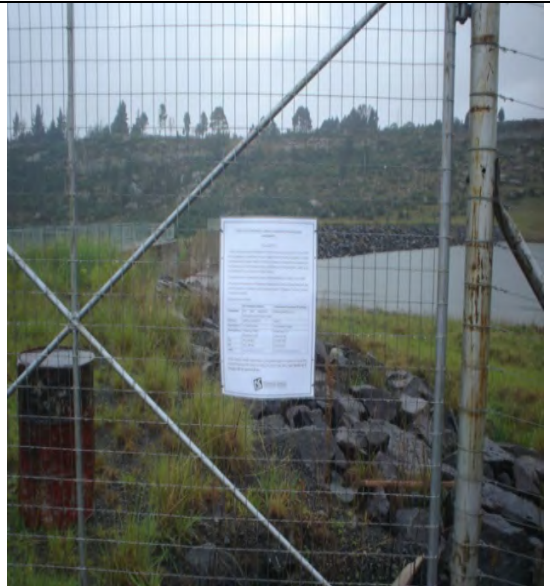
Photo2: View of the site advert and dam with granite stone gabions in the background.
