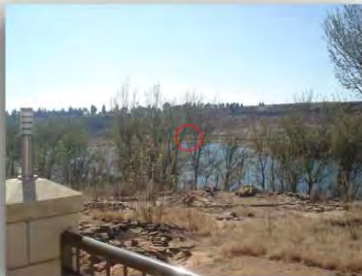
VIEW TOWARDS EXISTING DAM WALL WITH HYDRO IN POSITION STANDING ON THE 1ST PATIO OF THE SECOND UNIT FROM THE WEST
