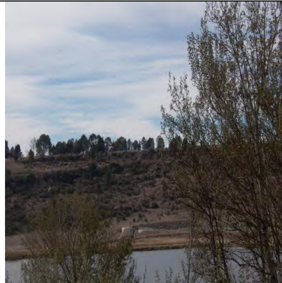
Photo 28: View of Boston A Dam weir from new residential development site.
