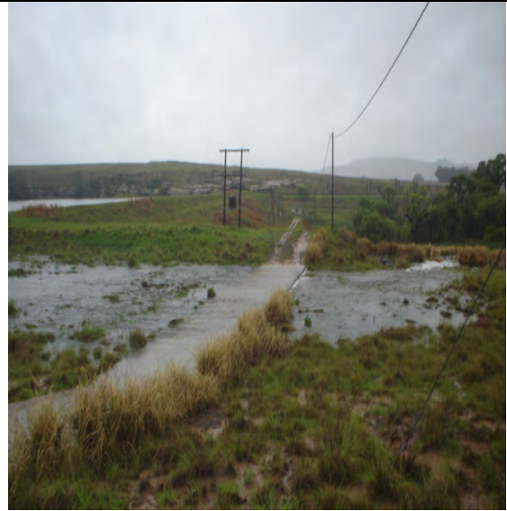
Photo 6: Private dam on adjacent farm overflowing the S217 dirt road.
