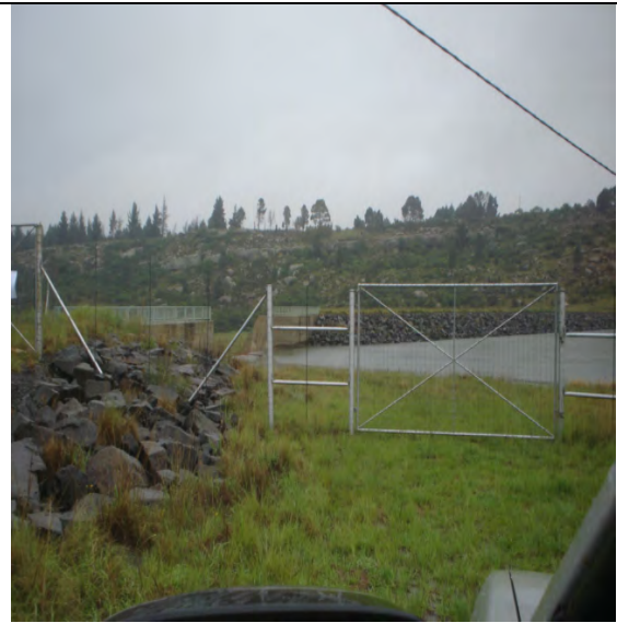
Photo 10: View of granite rock and gabions utilised for erosion protection.
