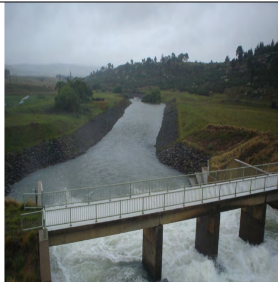
Photo 4: The only bridge providing access to the site on the north eastern bank of the Ash River. This 5 tonne bridge would not be able to support heavy equipment, machinery and construction vehicles.
