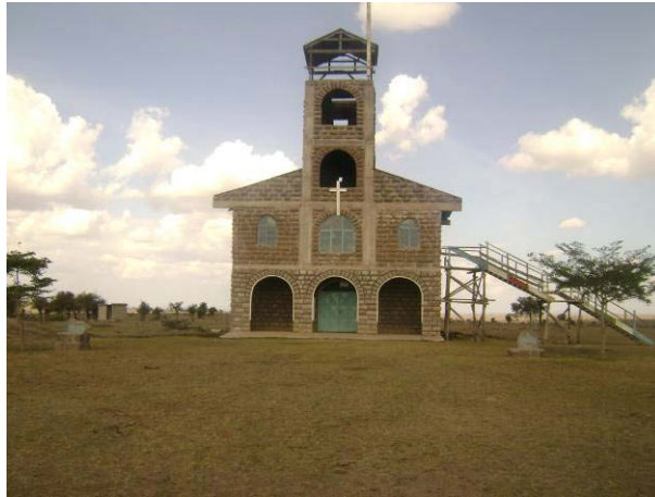
Fig.5.3: AIC church neighbouring Isinya substation at Kajiado district
