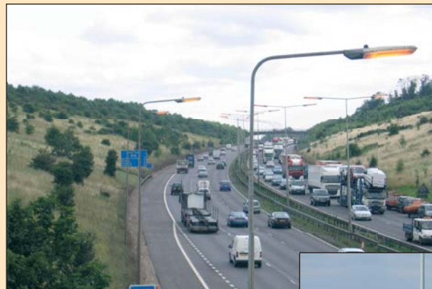
Existing congestion at Nags Head Lane on M25 Junction 28
