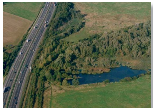
Example of drainage treatment measures at Ockendon
